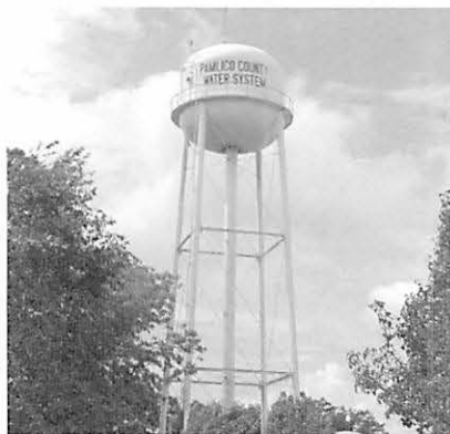
An improved water system is a sign of progress for Bayboro.
