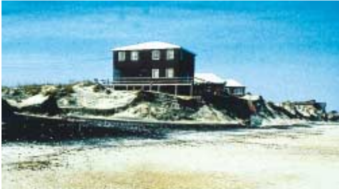
Photos 4 and 5: Although dunes provide storm protection, they aren't effective in preventing long-term or other types of chronic erosion.
