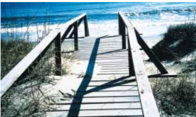
Photo 17: This is a good example of an elevated walkway with handrails.
