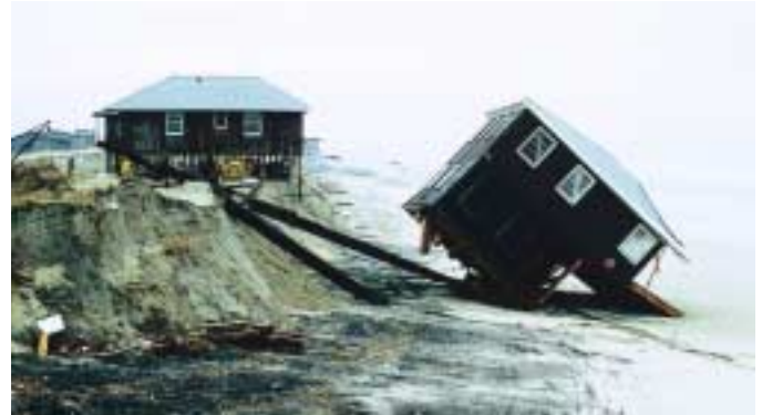
Photos 4 and 5: Although dunes provide storm protection, they aren't effective in preventing long-term or other types of chronic erosion.
