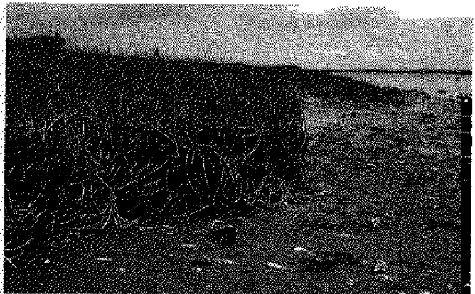
Figure 6. Undermining of a marsh in Carteret County.
