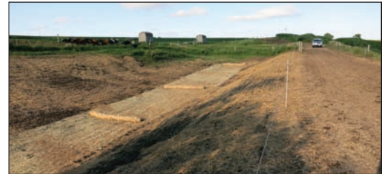
Figure 13a and b: Wood fiber blankets. Credit: Lawn and Driveway Service, Inc.
