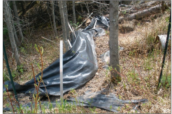
Figure 25: Remove silt fence when vegetation is established
