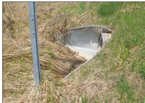
Figure 8: Most efficient, apron inlet
