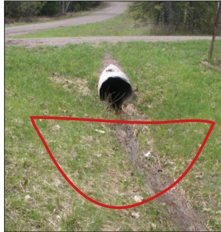
Figure 35: Example of a stable ditch shape
