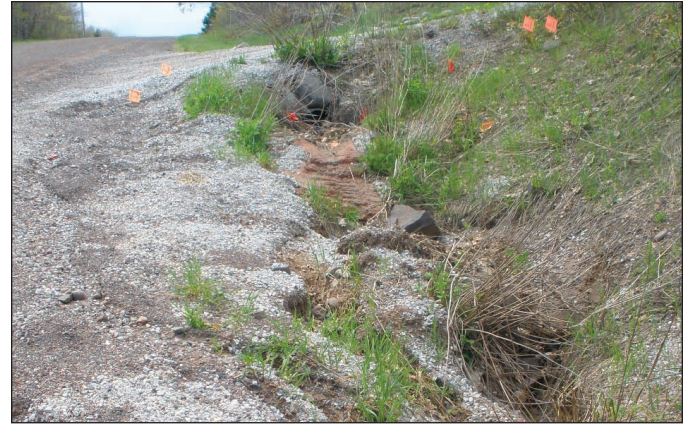
Figure 3: Unstable ditch
