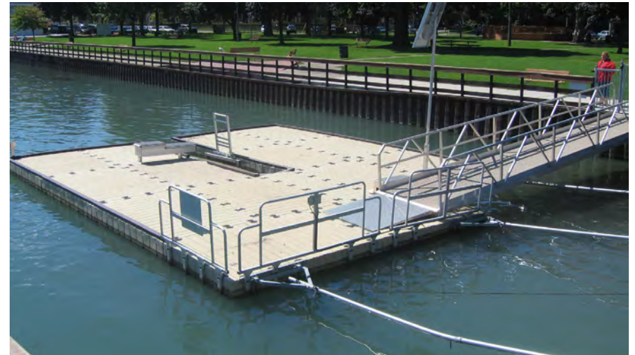
A solar-powered accessible launch in Wyandotte raises and lowers paddlers into the water.
