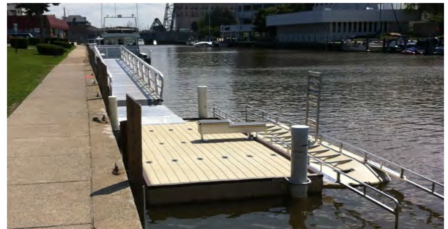
Depending on the physical limitations of your launch area, the gangway from the shoreline to the accessible launch may be quite extensive. This example is in Port Huron.
