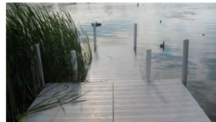
Launches on inland lakes should be located in protected areas with little or no erosion problems and minimal exposure to wind and currents.
