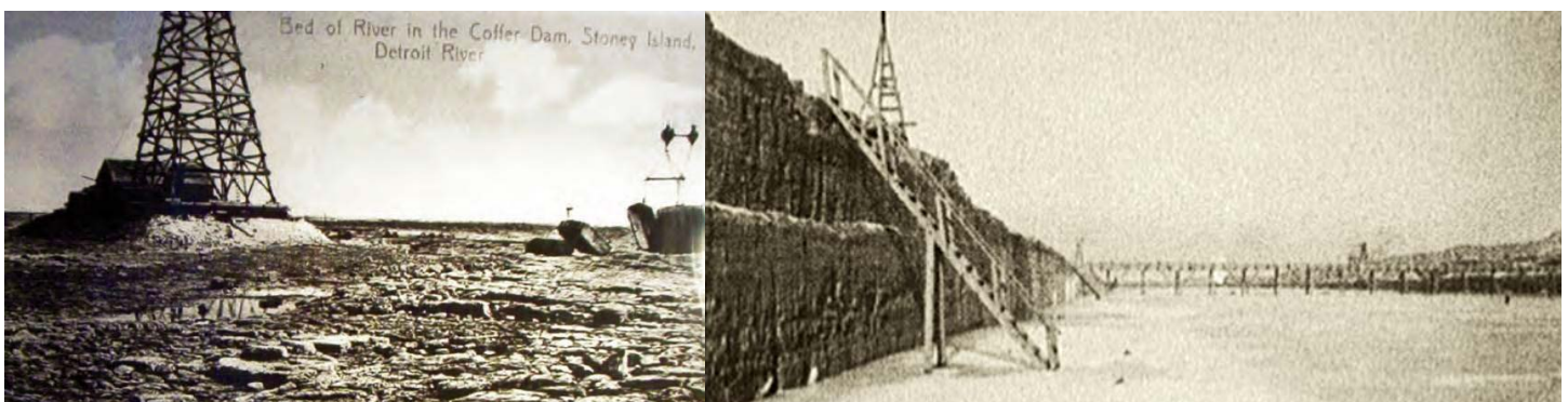
Figure 5. Historical photographs of the construction of the Livingstone Channel showing the limestone reef, dewatered, before and after blasting to deepen the channel.
