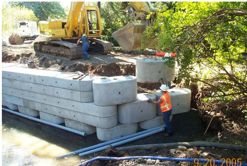
Precast concrete bridge abutments
