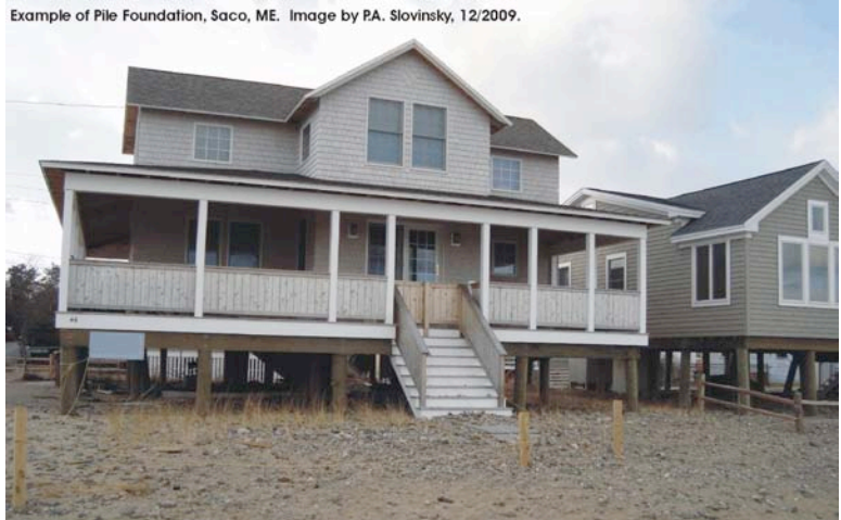
Example of Pile Foundation, Saco, ME. Image by P.A. Slovinsky, 12/2009.
