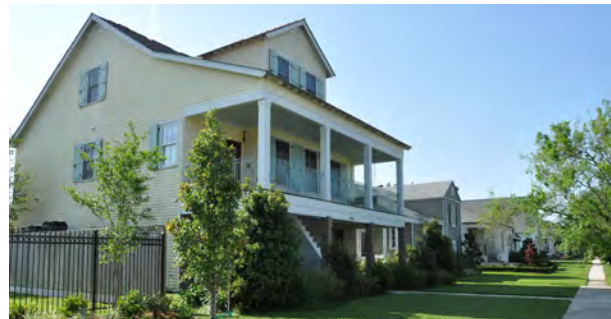
Neighborhood-scale design guidelines can help to retain the aesthetic qualities of a street while reducing risk.
