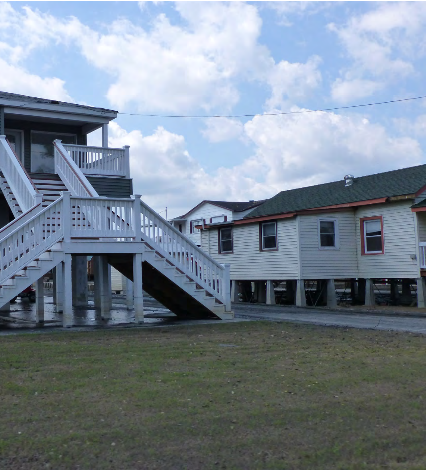
Elevating homes is a common approach used in Louisiana to reduce long-term costs associated with flooding.
