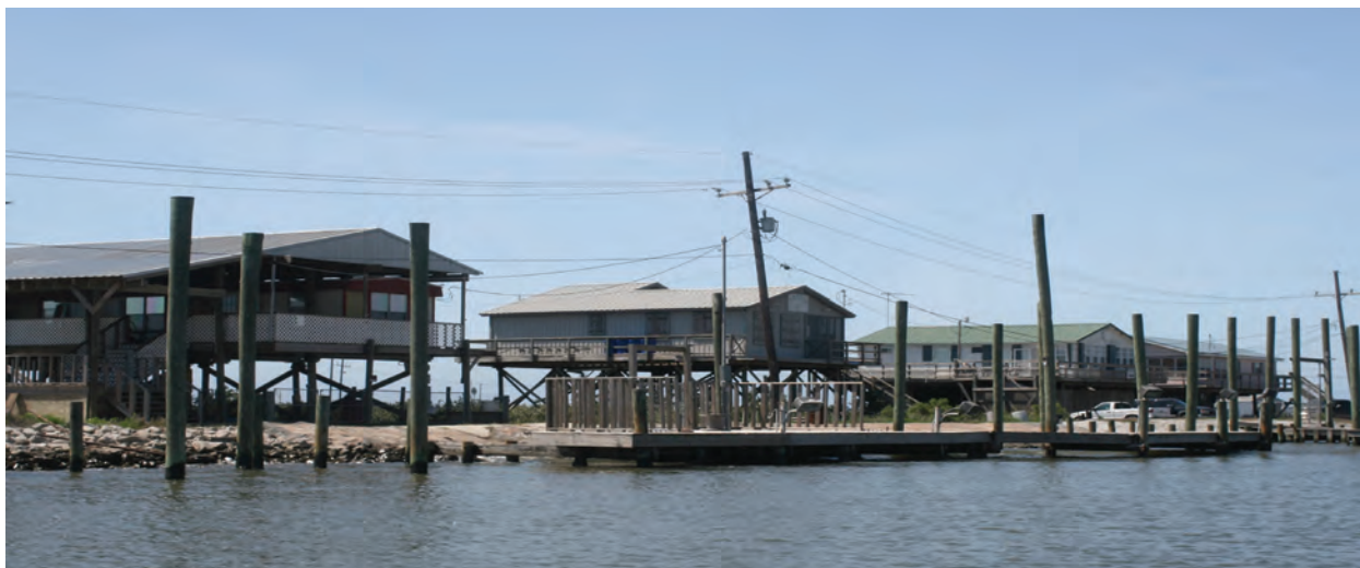
Elevated structures in southern Louisiana are one type of accommodation to adapt to sea level rise and increasing storm surge.
