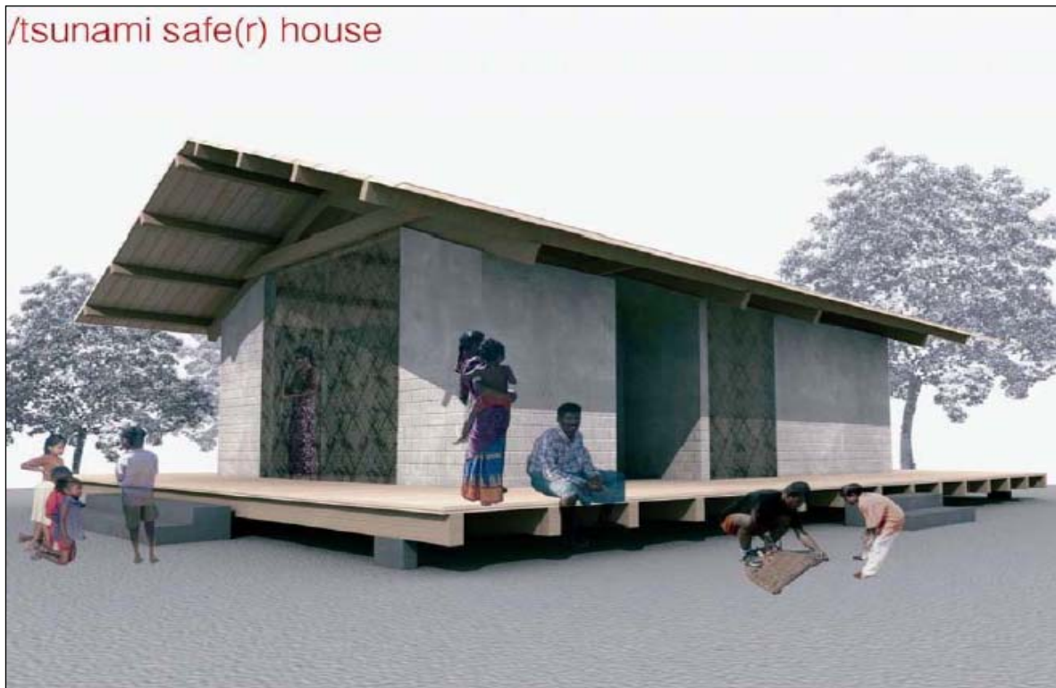
Figure 6-9 - Elevation on Piers and Columns to Address Flooding. Residential structures have been designed for Sri Lanka, using local materials and a modular design – From Dr. Carlo Ratti - MIT – Senseable City Laboratory, Boston, Massachusetts. Such a design is more economical and suitable for structures subject to flooding.
