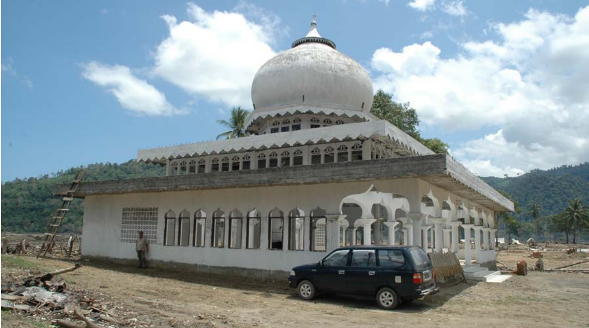
Figure 6-7 - Mosque at Jantang. This mosque was one of the few structures in the surrounding area that survived the tsunami inundation. Villagers climbed onto the upper floors to escape wave inundation. Again the concrete open framework that vented water played a role in allowing the structure to survive.
