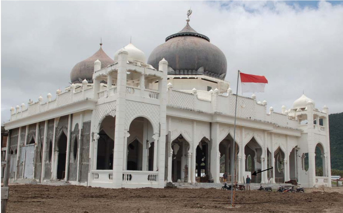
Figure 6-6 - Mosque at Lhok Nga. Many mosques in Indonesia were able to survive, despite the extreme wave height, even though all structures around them were destroyed. This is attributed to the concrete structure and open walls that allowed entry and exit water to vent through the structure. Note person at base of pole for scale. The water level was at a minimum 12 meters, or near the top of the first level. Mosque was about 800 meters from the shoreline. 26 Reports by interviewed survivors indicate water levels may have been higher.
