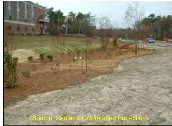
Infiltration Basin (During Installation)
