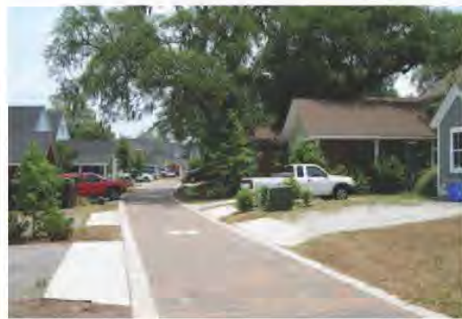
Sustainable technologies like the pervious paving above blend with old oak trees in this green development. Photo credits Southeast Watershed Forum.
