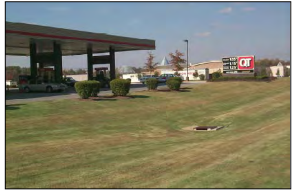
Filter Strip Around the Perimeter of a Parking Lot (Source: Atlanta Regional Commission, 2001)
