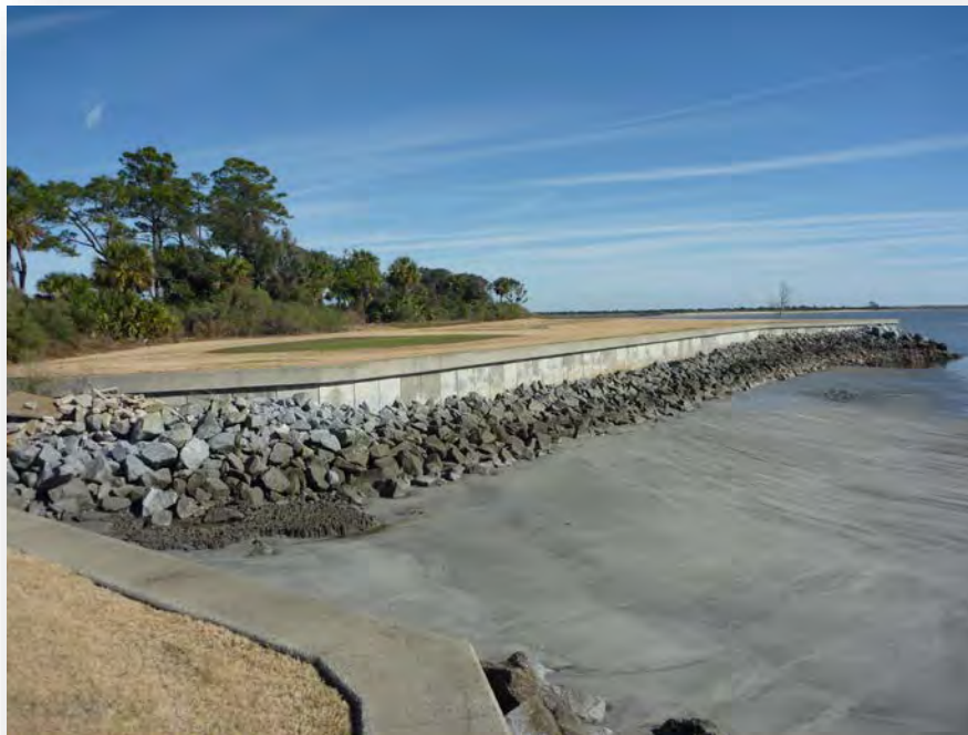
Typical Concrete Seawall, Source: Dr. Clark Alexander
