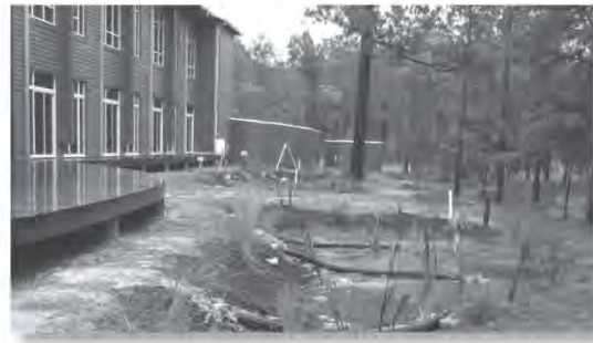
Researchers from Clemson University have recently designed, installed, and are currently studying water retention capacity and performance of bioretention cells at their new Baruch Institute facility in Georgetown, S.C. Photo/Clemson University
