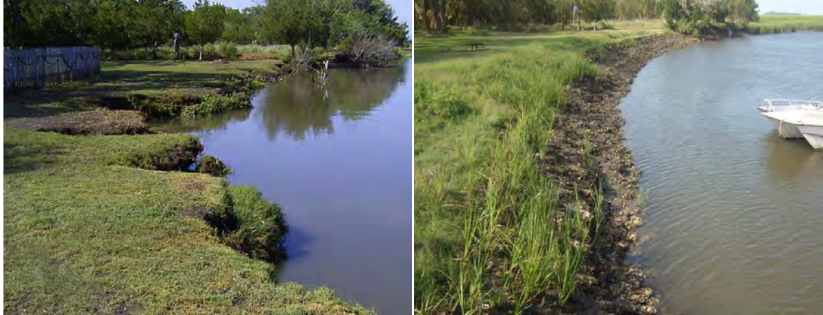
Ashantilly River - Before & After Stabilization. Source: Jan Mackinnon
