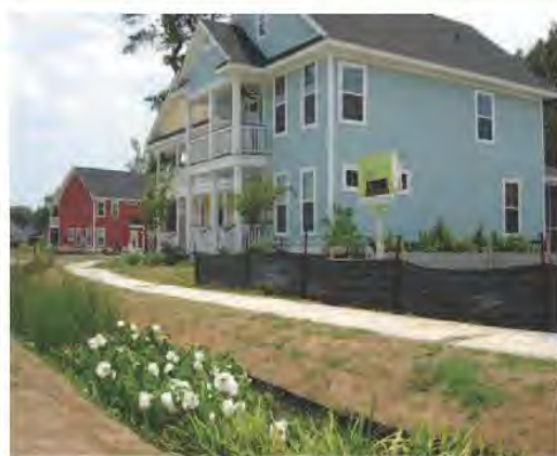
Bioswales enhance water infiltration into the soil, reducing runoff. Photo credits Southeast Watershed Forum.
