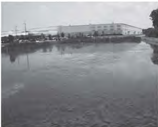
Stormwater ponds are designed to collect and concentrate pollutants and can promote algal blooms, such as these found in a pond in Berkeley County, S.C. Photo/SCDHEC-OCRM
