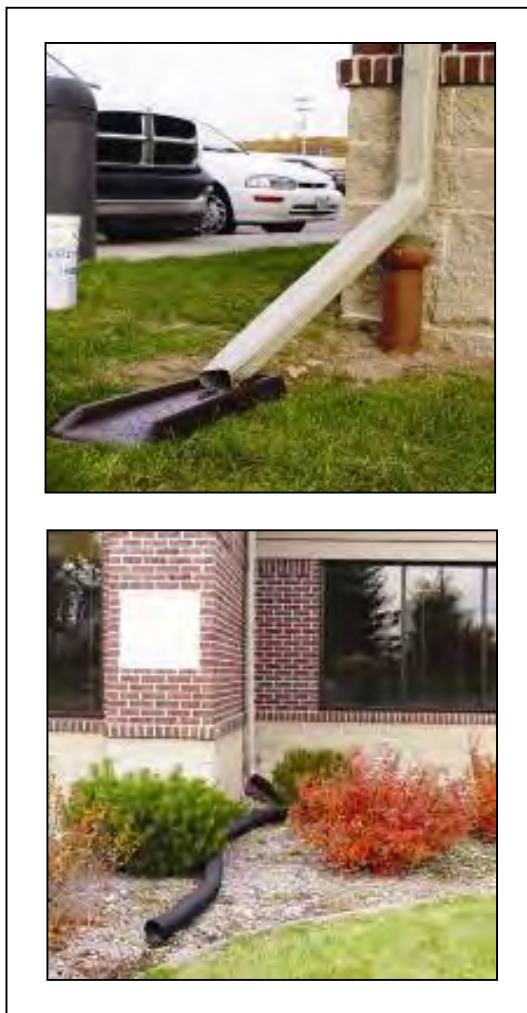
Simple Downspout Disconnections to Pervious Areas
