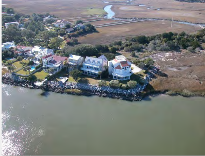
Typical Coastal Development with Structural Stabilization Measures (Bulkheads/Rip Rap Revetment). Source: Dr. Clark Alexander
