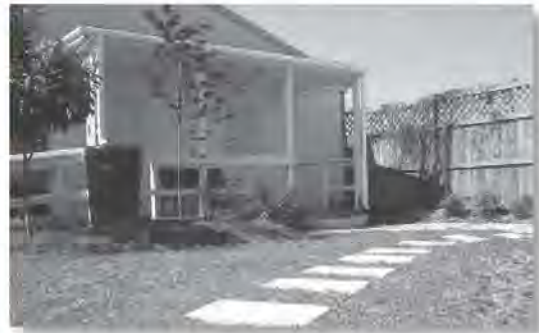
The Clemson Extension Carolina Yard constructed at the Charleston Exchange Park incorporates the use of pervious pavers, pervious walkways, a rain barrel, and a rain garden to educate the general public on the site-scale use of LID practices. Photo/USC
