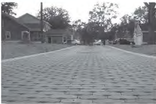
University of South Carolina researchers are studying the cumulative impacts of LID practices (e.g., bioretention swales, pervious pavers, pocket parks, pervious walkways) at Oak Terrace Preserve in North Charleston, S.C. Photo/City of North Charleston
