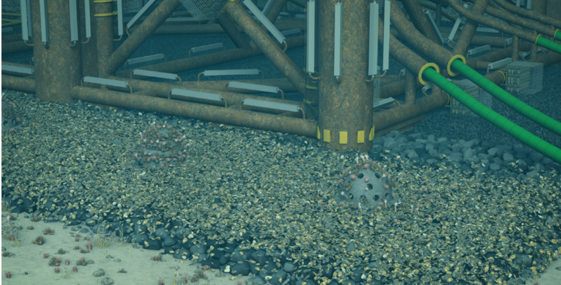
Figure III: Visual representation of the scour protection eco-cable crossing. Image courtesy of TenneT.
