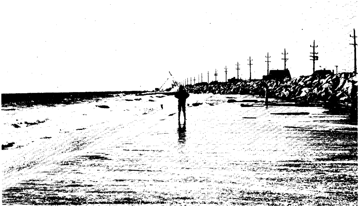
Figure 28. Rip-rap seawall, Sandy Hook, 23 September 1960. (Photo by W. Yasso)
