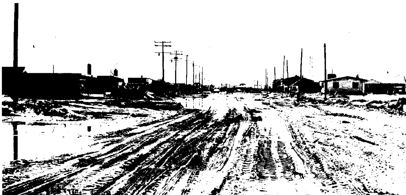
Figure 25. Sand deposits on Long Beach Island road one week after great Atlantic coastal storm, 16 March 1962. Note the partly destroyed house on the left. (Courtesy of NJ Department of Environmental Resources)
