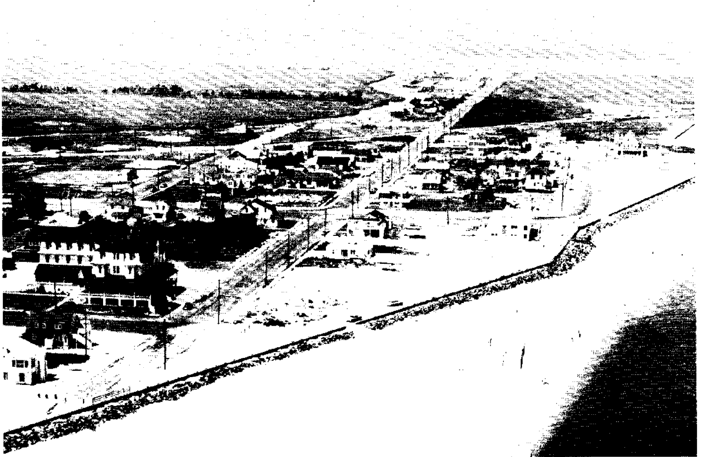
Figure 27. Revetment and timber bulkhead at Avalon, NJ, low tide, August 1963. (Photo by E. Miller, courtesy of mayor's office Avalon, NJ)
