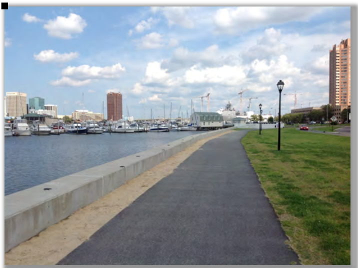
Figure 3.10.3:6 - Portsmouth's newly elevated bulkhead and bicycle/pedestrian path
