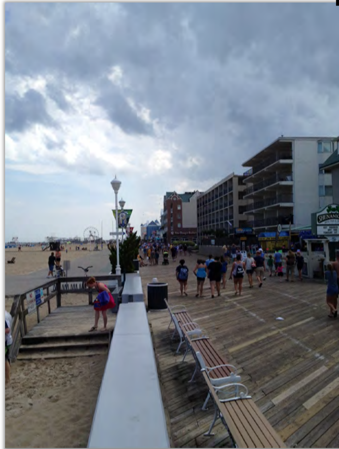
Figure 3.9.1:2 - Ocean City's boardwalk and reconstructed seawall
