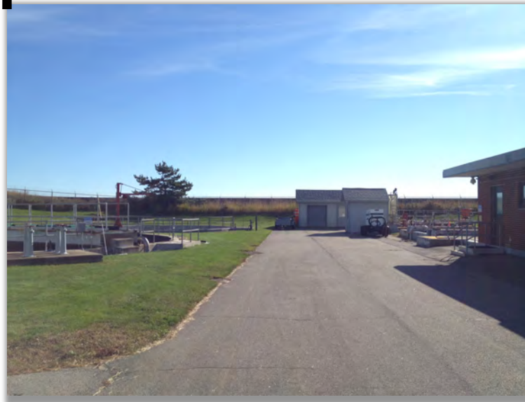
Figure 3.1.1:1 - Ogunquit's treatment plant is located just over the primary dune
