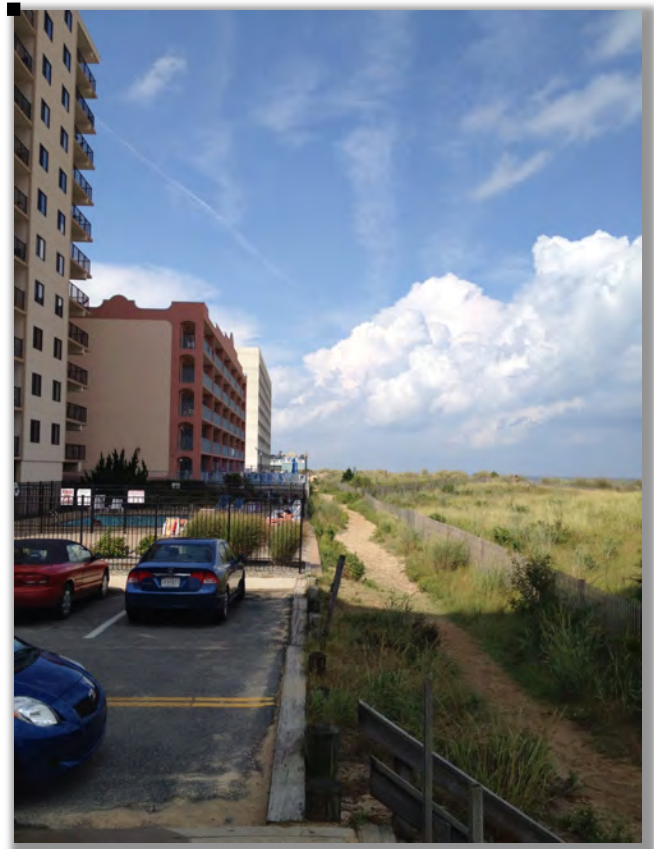
Figure 3.9.1:1 - This image clearly depicts Ocean City's build-to line and reconstructed dune enabled by the TDR program and beach replenishment project
