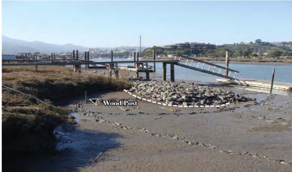
Figure 9. Photograph showing "outflanking", or erosion at the end of a marsh sill, which is typical of coastal structures over their design life (ESA 2017). The wood post shows the distance between the eroded marsh edge and landward side of the sill.
