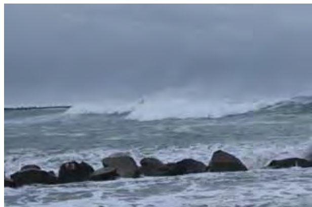
North Jetty inundated by storm waves
