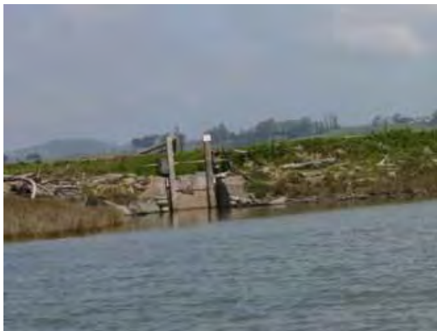
Many tidal sloughs are controlled by tidegates
