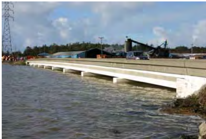
Highway 255 bridge at Mad River Slough
