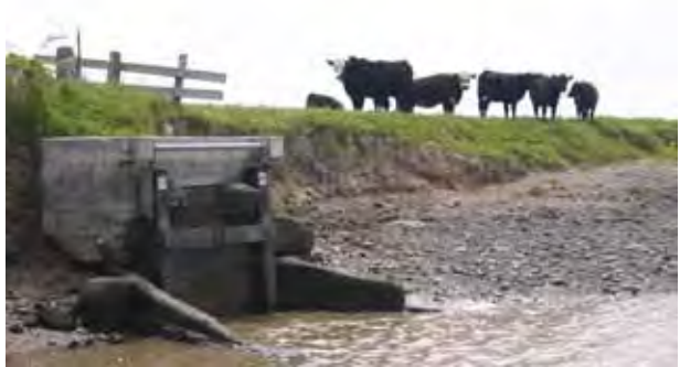
Levee without hardening
