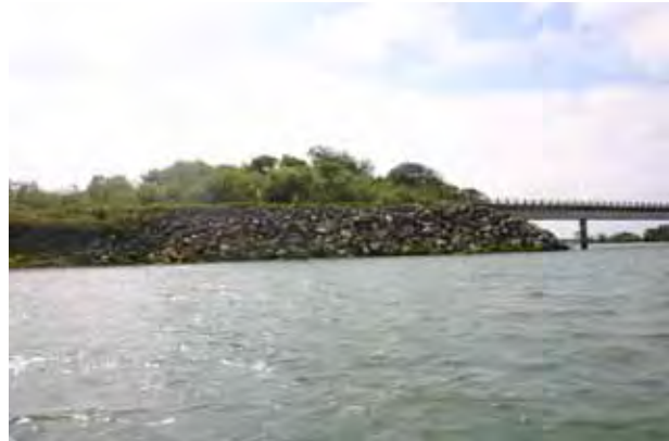
Levee with rip rap at Cock Robin Island
