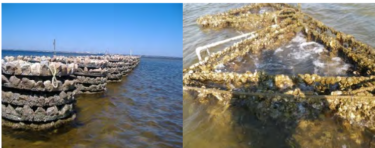
Figure 2- Two designs of breakwaters. A modified version of the Ecosystem by Reefmaker, David Walters -Orange Beach, Ala., (left) Reefblk by Coastal Environments Inc., Mark Gagliano- Baton Rouge, La. (right)
