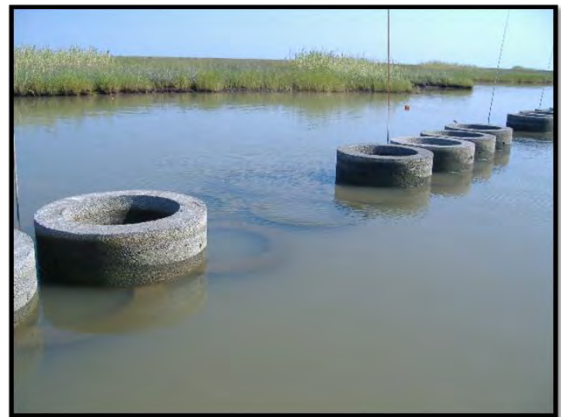
Figure 1. Nature Conservancy emplacement of Oysterbreak™ rings in Vermilion Bay, La., added habitat and reduced erosion.
