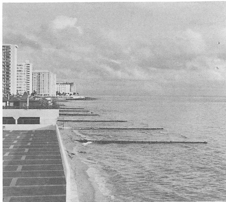
Fig. 3.7. The "old" Miami Beach, 1972. The principal reason that the beach disappeared in Miami Beach may simply be that buildings were built virtually out on the beach. Photo by Orrin Pilkey, Jr.
