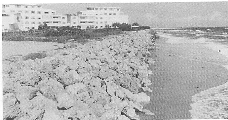
Fig. 3.17. The revetment at Ocean Ridge, South Palm Beach. Photo by Dinesh C. Sharma.
