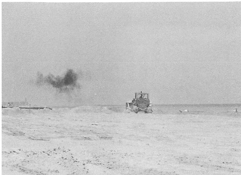
Fig. 3.3. Molding sand recently pumped up on a beach with a bulldozer, Lauderdale-by-the-Sea. Photo by Bill Neal.
