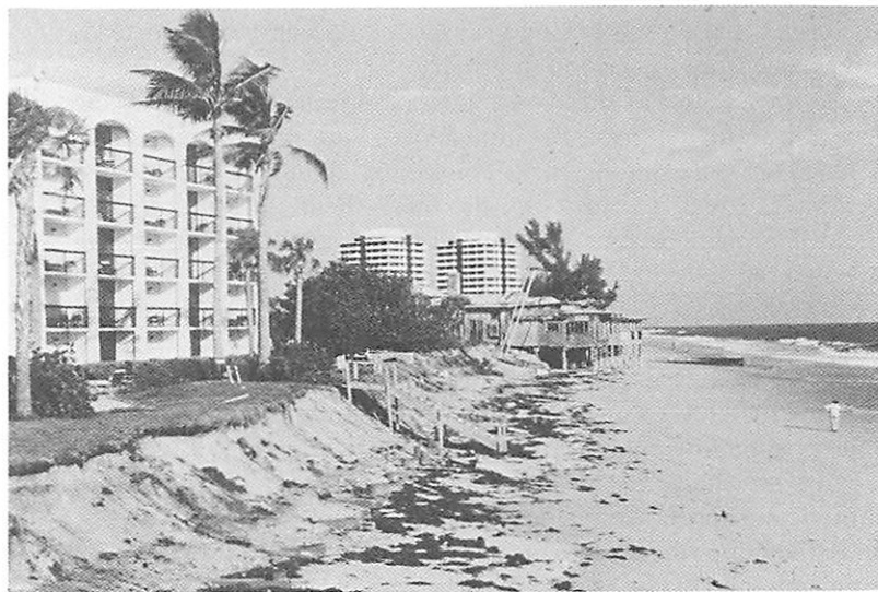
Fig. 2.12. Beach erosion is about to catch up with this condo and has already caught up with the house down the beach. This is a low-tide scene from Vero Beach, looking north. Photo by Dinesh Sharma.
