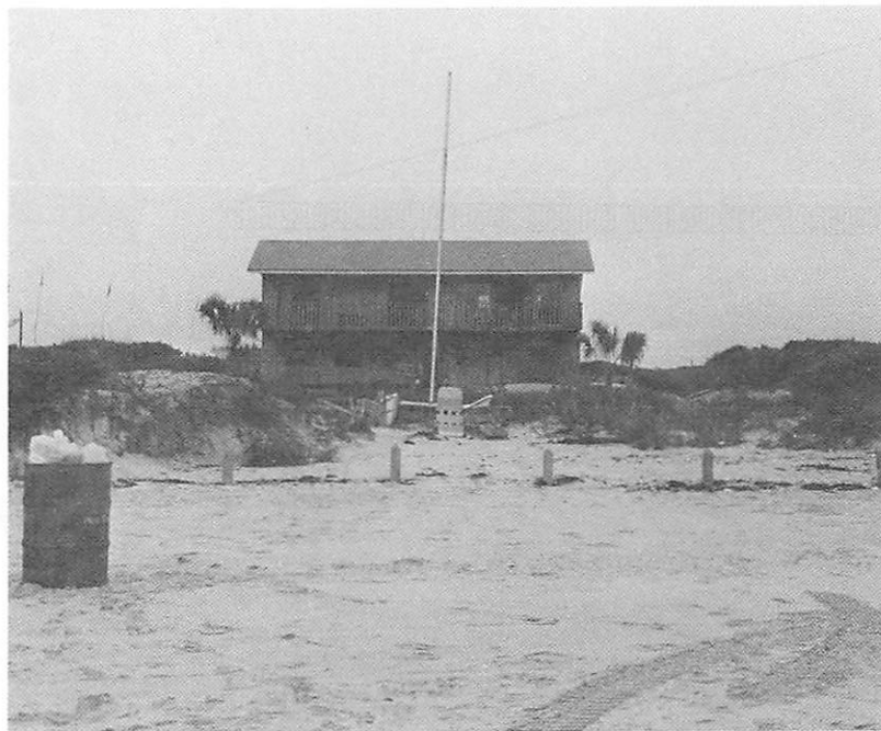
Fig. 4.21. The primary dune was removed to site this house in Wilbur-by-the-Sea. Photo by Barb Gruver.
