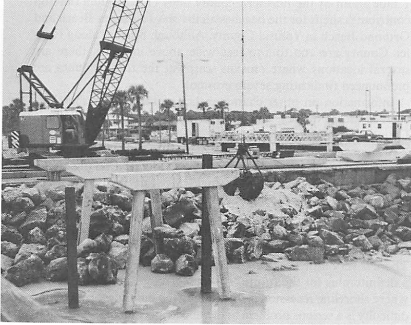
Fig. 4.15. Seawall reinforcement, St. Augustine Beach. Photo by Bill Neal.
