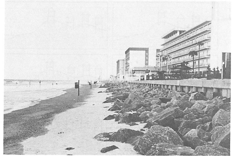
Fig. 3.15. Neptune Beach seawall and revetment. Photo by Dinesh C. Sharma.
