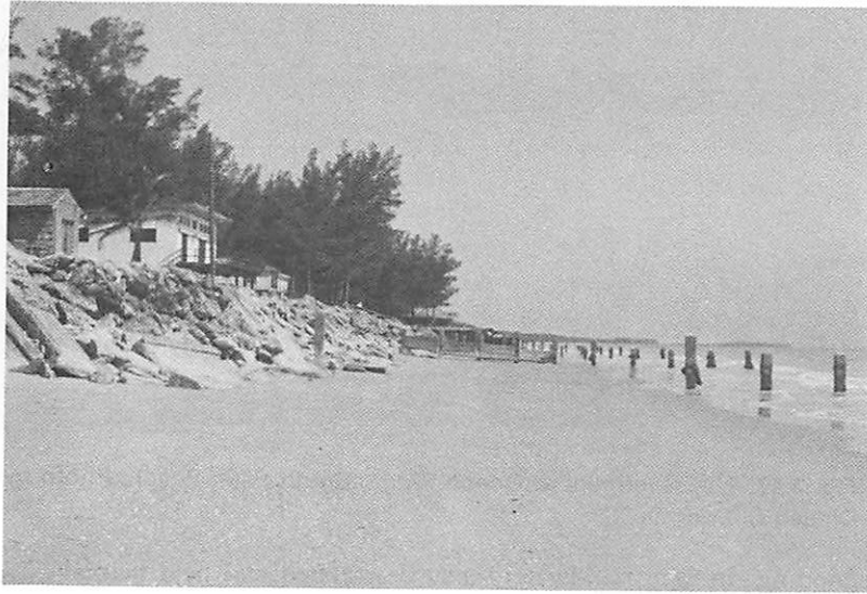
Fig. 3.14. Revetment at the north end of Jupiter Island. Columns in the water are probably remnants of destroyed groins. Photo by Barb Gruver.
