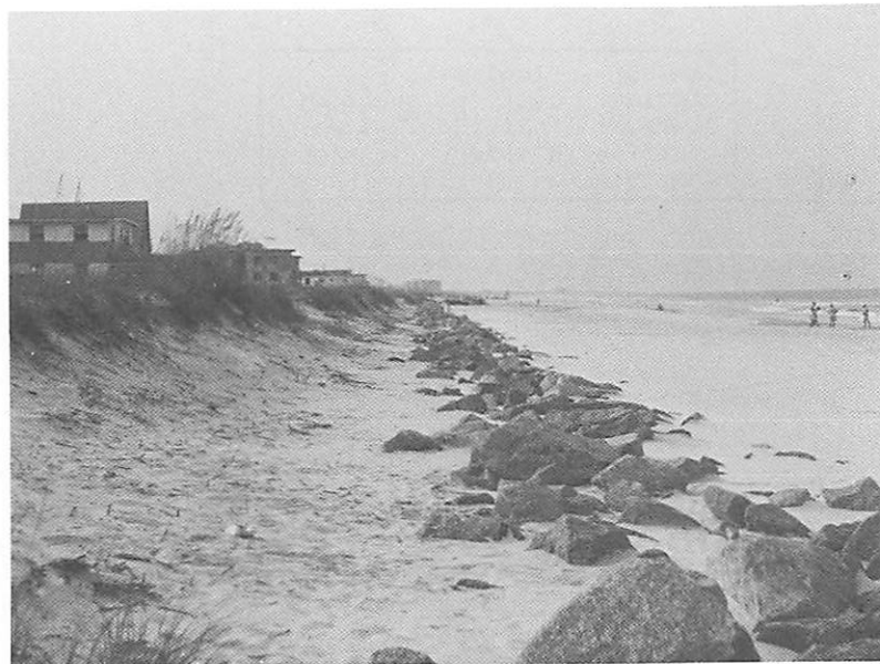
Fig. 4.9. A small row of rocks has failed to halt shoreline retreat at American Beach, Amelia Island. Photo by Bill Neal.
