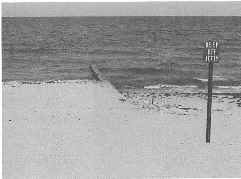
Fig. 3.10. A small groin incorrectly labeled as a jetty. North is to the right. Photo by Bill Neal.
