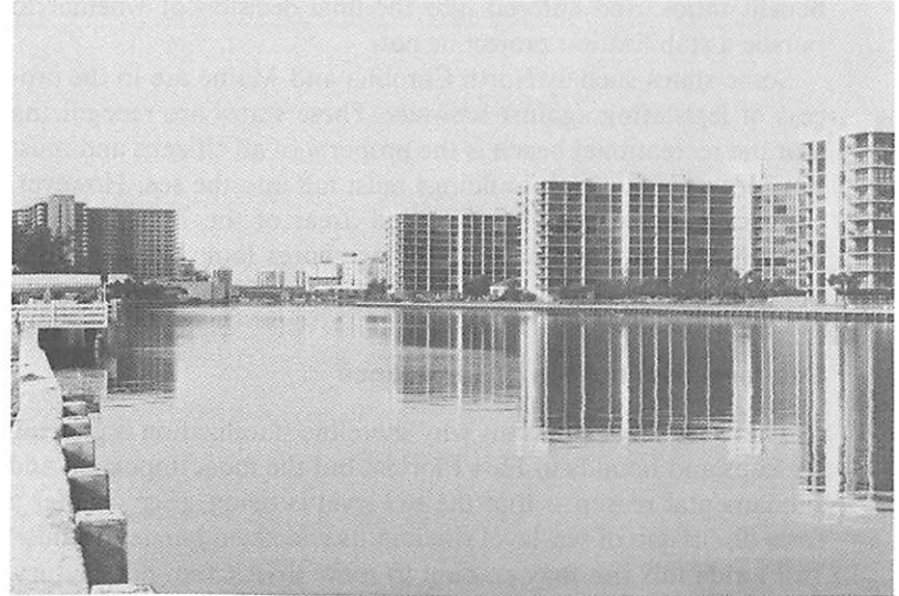
Fig. 3.18. Most of the heavily developed Florida islands are completely bulkheaded on the back side. This example is in Hallandale Beach. Photo by Orrin Pilkey, Jr.
