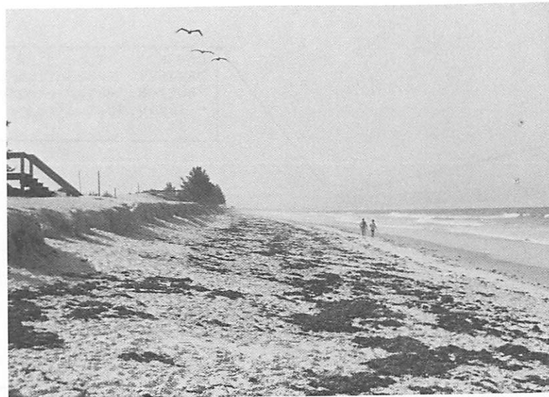
Fig. 4.32. Erosion scarp on the beach at Patrick Air Force Base. The nourished beach is disappearing rapidly here.
