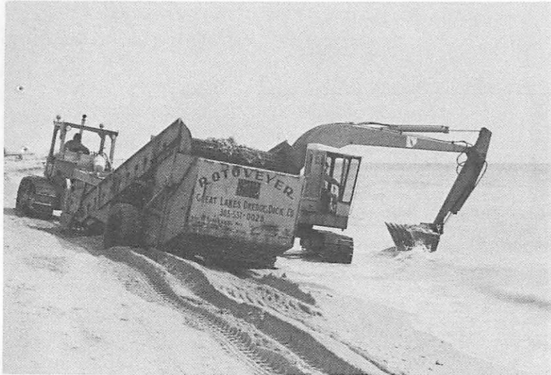
Fig. 3.5. Removing coral fragments from a replenished beach to increase the "swimmability." North of Hollywood Beach. Photo by Bill Neal.
