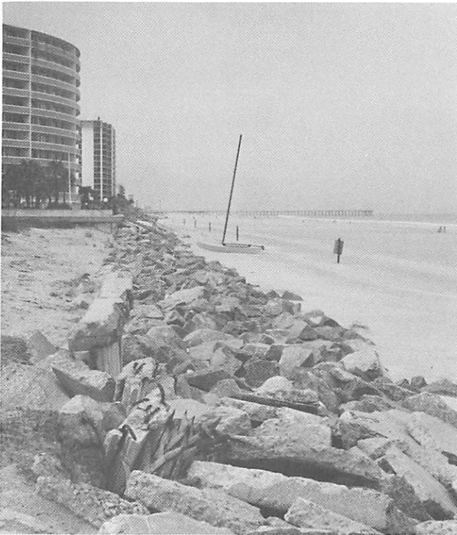
Fig. 4.13. Revetment in front of a destroyed seawall, Jacksonville Beach. Photo by Bill Neal.
