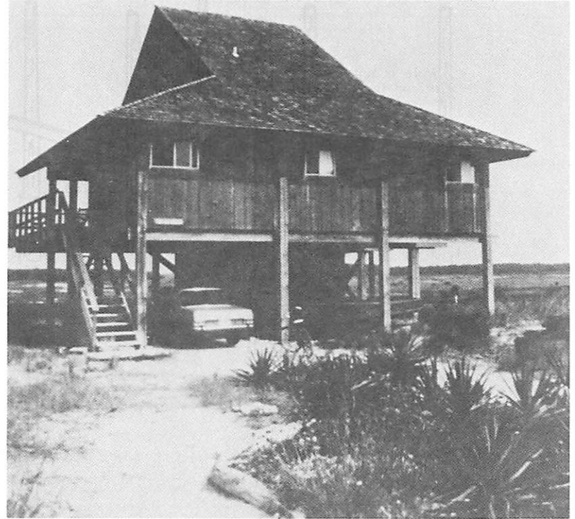
Fig. 6.4. Pole house, with poles extending to the roof. Extending poles to the roof, as shown in this photograph, instead of the usual method of cutting them off at the first floor, greatly strengthens a beach cottage. Photo by Orrin Pilkey, Jr.
