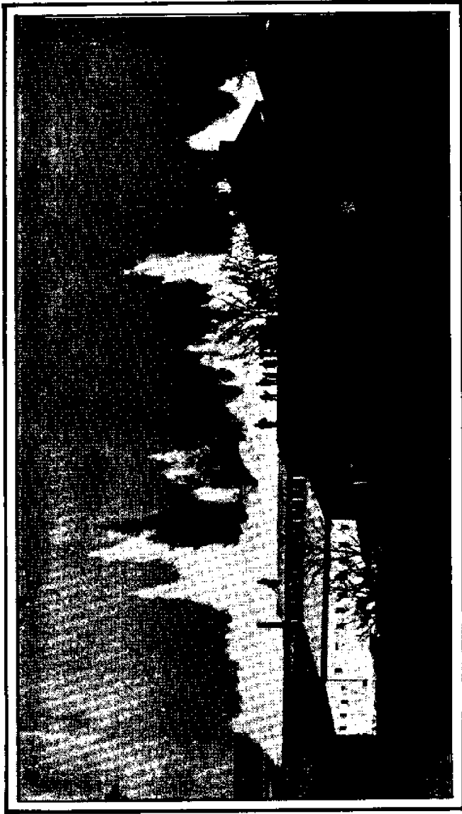
Figure 15 Clearing of the East River Channel, now called Hell's Gate was one of the US Army Corps of Engineers' first major operations. Tunnels were dug from land out under the reefs and then filled with explosives. The resulting explosions, which destroyed Flood Rock and Hallett's Point Reef, were among the largest man-made explosions to that time, 1885. Source: Museum of the City of New York.
