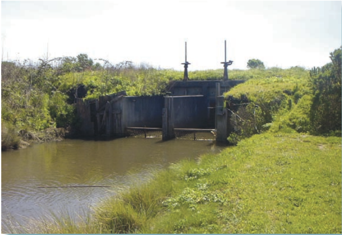
Figure 24. Tide gate separating Eureka Slough, Humboldt Bay, Humboldt County, California, and the drainage ditch that parallels California State Highway 101. The drainage ditch is in the foreground.
