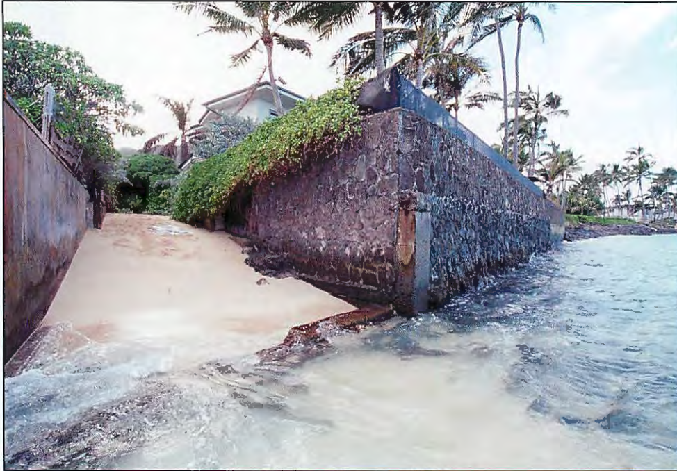
Figure 1-7 – Shoreline Public Access – An increasing number of public access ways required under State & county law no longer lead to recreational areas, but walled fortifications. Waves break against the wall and run up the access way, eliminating access along the shore (horizontal access) and restricting ingress to the shore (vertical access).
