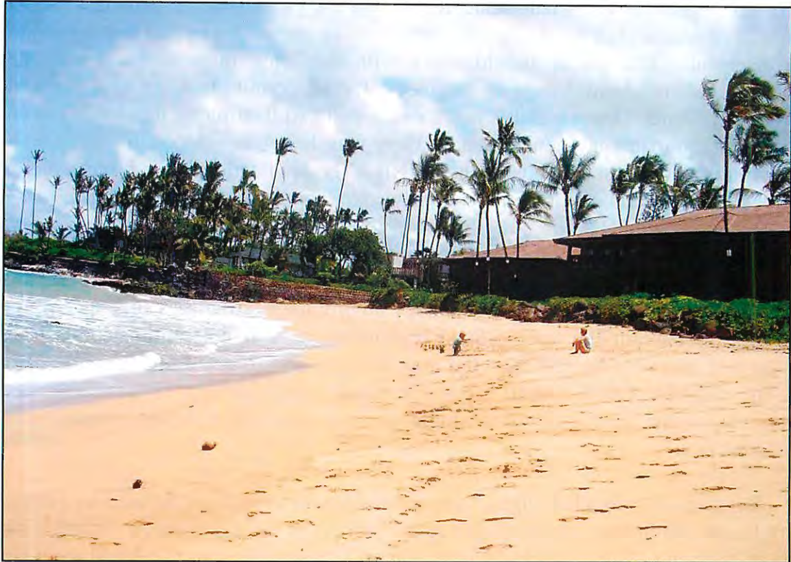
Figure 12-5 – Sand Replenishment, Maui – Inland dune sand placed on the beach has created a buffer zone that protected residents from high surf in the winter of 2001. During high wave activity, the sand created offshore bars that caused waves to break farther offshore. Photo by Barbara Guild, Maui.
