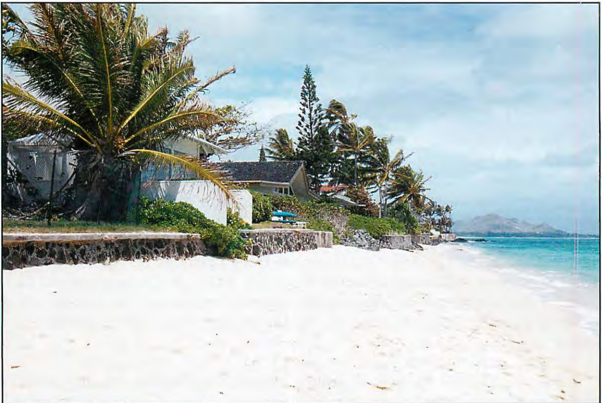
Figure 12-1 – North Lanikai, Oahu - Example of a shoreline hardened with a seawall, and a beach in front. Many beaches with a history of alternating erosion or accretion, or short-term erosion may not be lost in front of the hardened shoreline.
