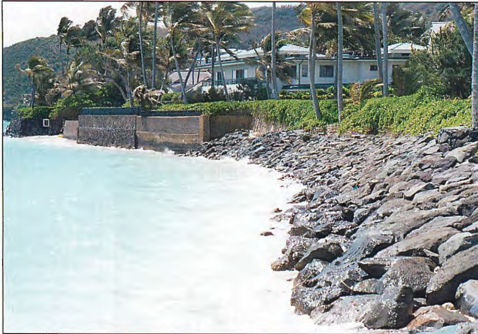
Figure 1-5 - Lanikai Beach, Oahu – Hardened Shoreline - Section adjacent to Figure 1-4 but facing southeast. Homeowners attempt to permanently fix the shoreline with seawalls and revetments. The beach is lost and there is reduced recreational value. Access along the shore is cut off. State resources are impacted.
