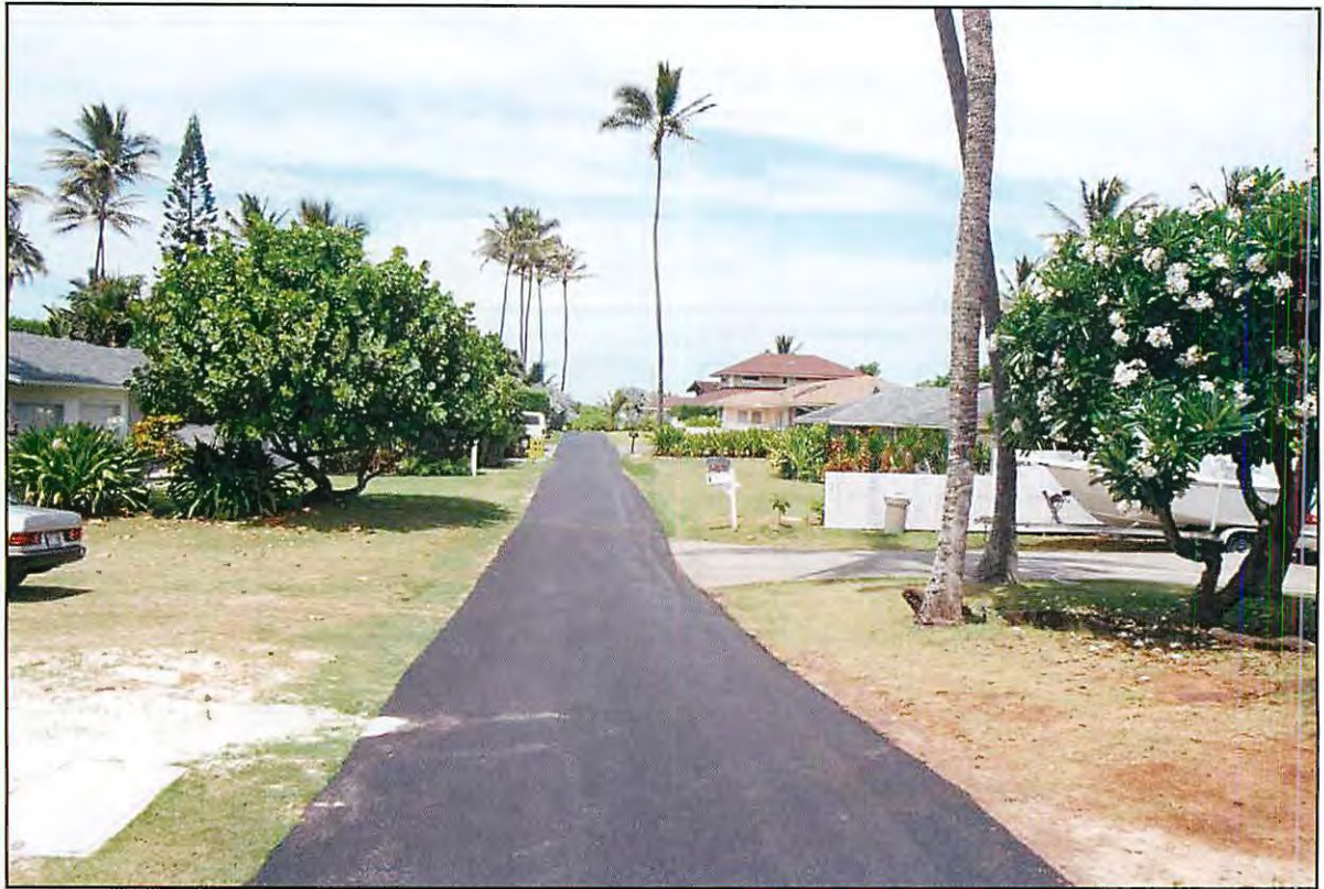
Figure 8-5 – Kailua Beach, Oahu – Feeder Roads - Example of a coastal lots being served with feeder roads perpendicular to the shore. Lots are deep and accommodate a sufficient setback (Figure 8-2). The ocean is in the background.
