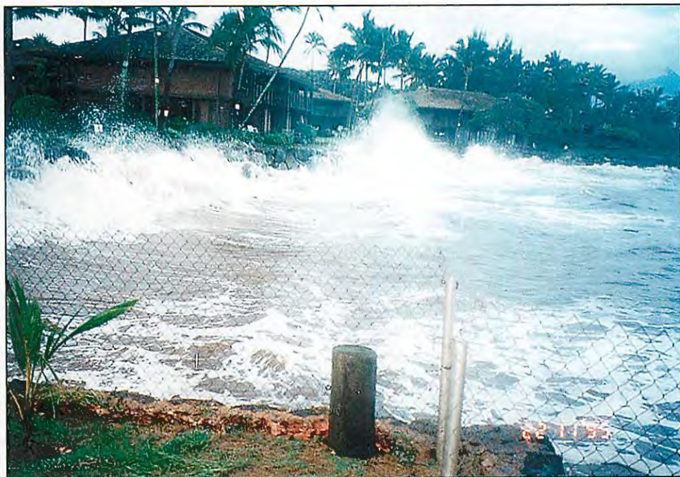
Figure 1-10 - November 22, 1995 Storm - Sugar Cove, Maui. With no beach in front of the boulder wall, winter waves impinge on the entire length of the wall. Buildings are inundated as waves crash against the hardened structures and reach the 2 nd story bedrooms. Photo by Barbara Guild, Sugar Cove, Maui.
