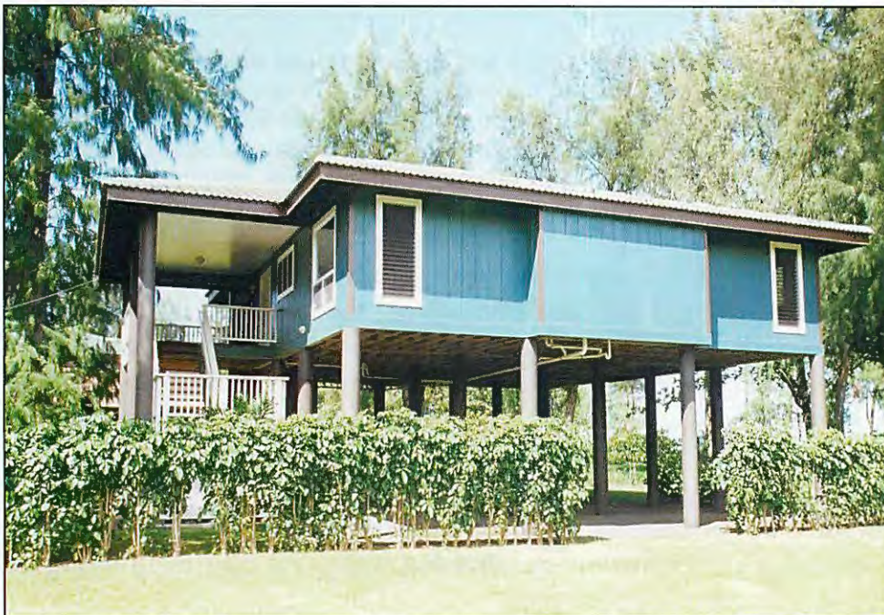
Figure 2-7 – House Above the Base Flood Elevation at Haena, Kauai - Many of the flooding issues associated with coastal storms, tsunamis or hurricanes can be addressed at Stage 7, by elevating the house so that the lower floor is above the 100-year flood water levels (i.e., the base flood elevation). A margin of safety can be built in by constructing a few feet higher than the BFE.
