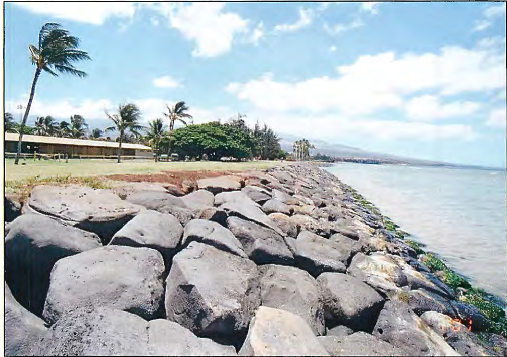
Figure 1-6 - Kalama Beach Park, Maui - Beach Park on Maui without a beach. A long stretch of shoreline is hardened with a stone revetment along a former beach area.
