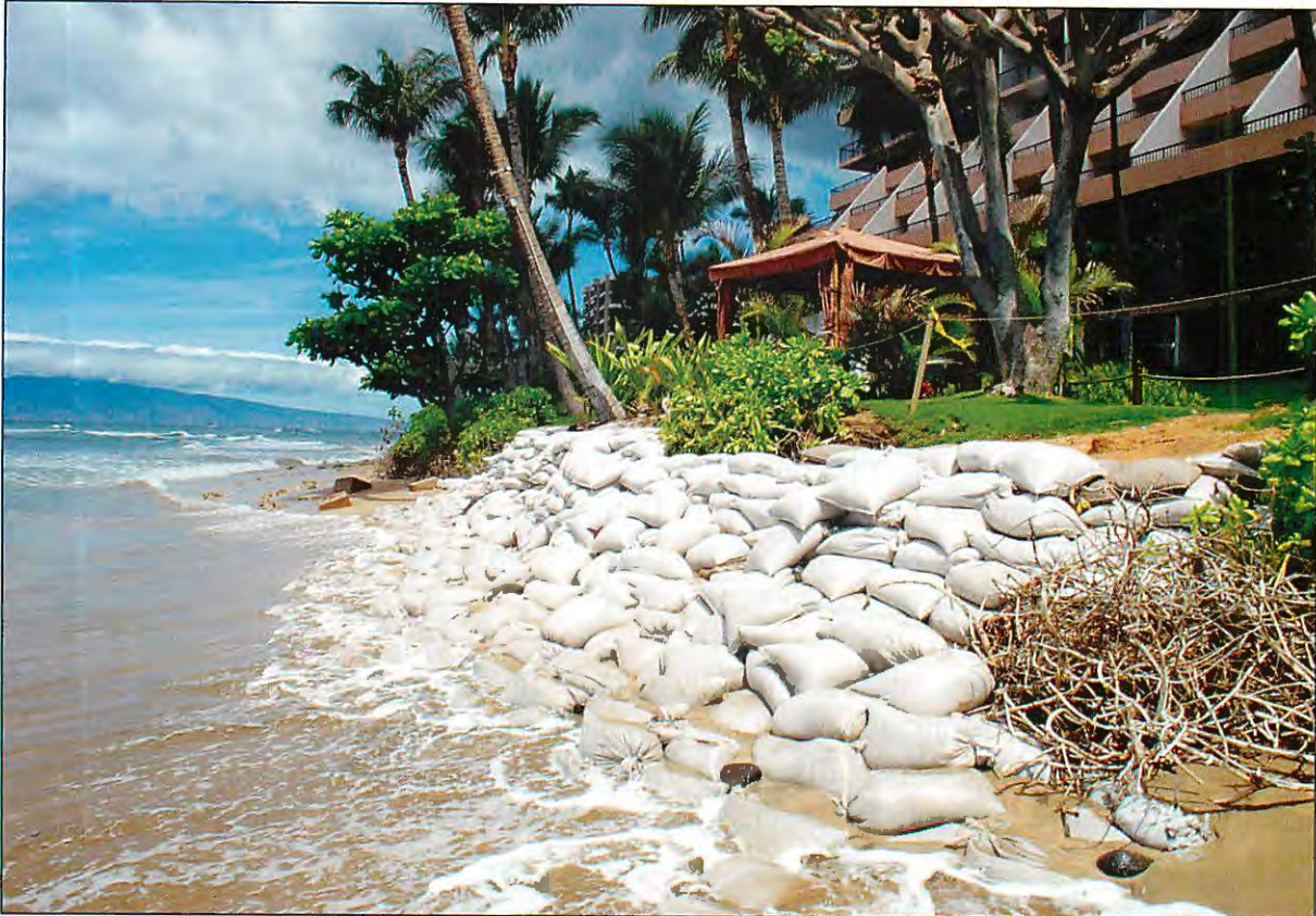
Figure 12-4 – Small Sand Bags for Erosion Control, Maui – Small sand bags are placed along this shoreline to protect trees and structures from erosion. The bags at Kaanapali have provided limited temporary protection as waves have eventually moved the bags along the shore.
