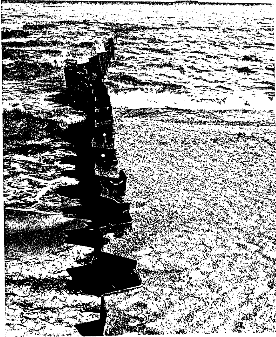
Figure 5-B Mixed sand and gravel beach accumulated on the updrift (east) side of a steel, sheet-piling groin at Crane Creek State Park, Ottawa County, Ohio; note coarse nature of beach material at crest of berm.
