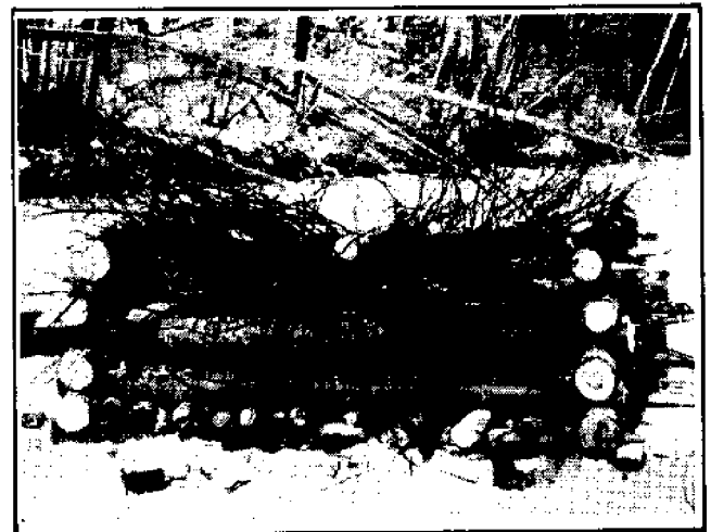
Figure 9. Wisconsin log crib being constructed on winter ice. Photo courtesy of Paul Brouha, Wisconsin Department of Natural Resources.
