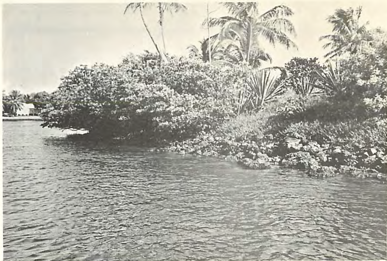
FIGURE 2. Riprap treatment of sloping banks
