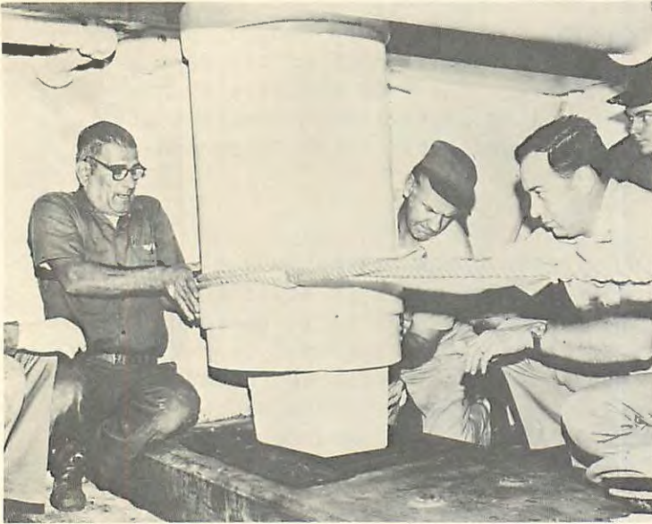
Stepping the mizzenmast - through three decks. The traditional coins, including a 1797 penny, have already been placed beneath the mast. The intensity of expression on all present is indicative of the care and precision needed to bring it off successfully.
