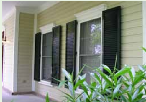
Figure 4-14. Colonial shutters made from durable extruded aluminum components add a traditional look to the home and provide effective opening protection. Source: Roll-a-way/QMI
