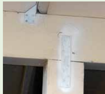
Figure 4-28. In this retrofit example, a hurricane clip attaches the roof structure to a horizontal ridge beam, which is in turn attached to the vertical post with a metal strap. This is an attempt to tie the load from the roof to the foundation, or create the complete load path connection. Note that these clips and straps are in the process of being painted. Source: Hurricane Protection Services.
