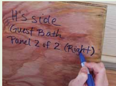
Figures 4-21 and 4-22. Not only is it necessary to install plywood opening covers correctly, it is also important to correctly label them and store them away from heat and humidity.
