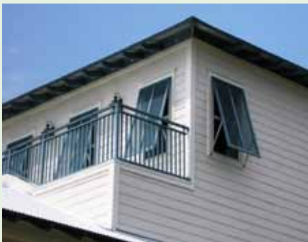
Figure 4-13. Bahama shutters made from durable extruded aluminum components add "Islands" flair to a home and provide effective opening protection. Source: Roll-a-way/QMI
