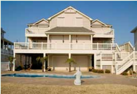
Figure 4-10. Coastal home protected with roll-down shutters on all windows and doors. The shutter is held in place by vertical guide tracks and can be deployed manually or with integrated electric motor. Source: Roll-a-way/QMI
