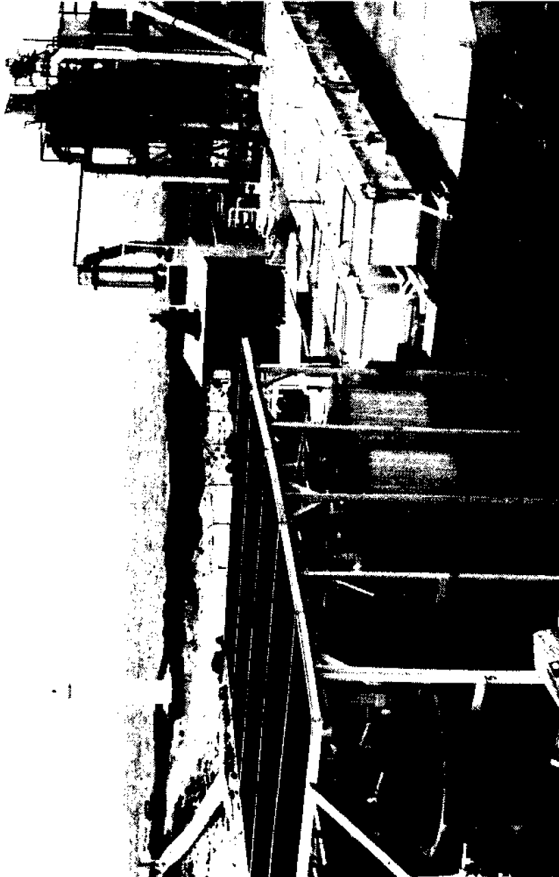
Figure 2. Experimental OTEC aquaculture facilities at NELH. The round fiberglass tanks on the lower left, covered overhead with shade cloth, were used for salmon and trout experiments. The rectangular tanks to the right of the fish tanks were used for nori tumble culture. The surface and deep seawater pipes on the left lead from the ocean between the lighthouse and the top of the fish tanks to the header tanks on the upper right.
