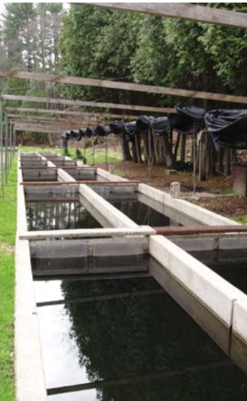
7.2 Concrete, parallel/series hybrid, single-pass raceway. Chris Hartleb
