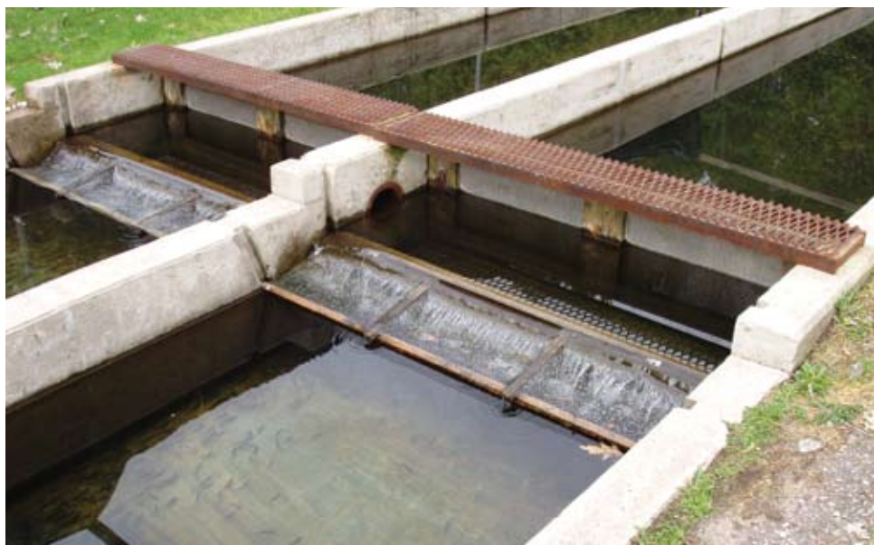
7.6 Splash boards and screening at the levee of a multiple series raceway. Chris Hartleb
