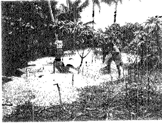
Filling on the north end of the island progresses. Note the sticks marking the squares. The ribbons on them indicate the level to which the squares will be filled.
