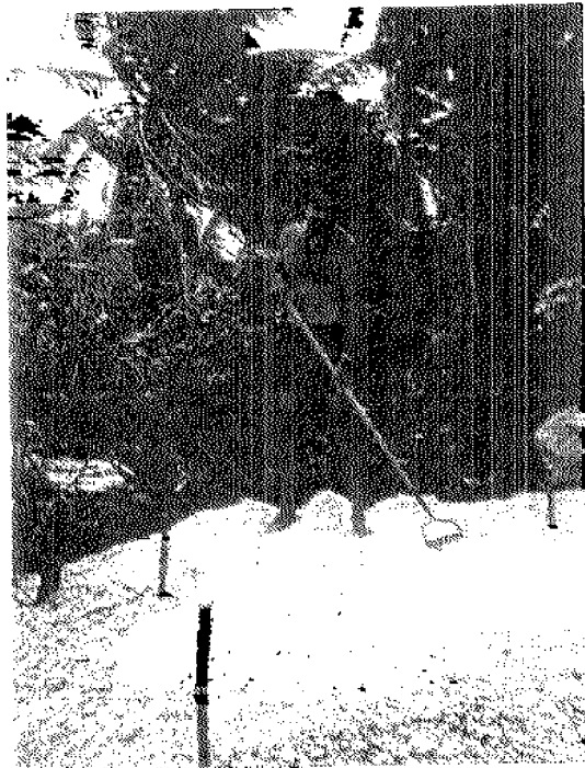
My job at the project site was to rake the filled material level with the ribbons on the top of the sticks. This insured that the reclaimed area would have a pleasing contour. In this photo, I am spreading the final layer of sand over the coarser gravel below.
