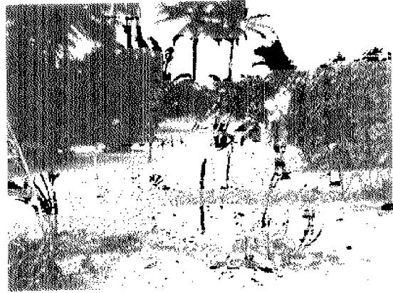
Filling on the north end of the island progresses. Note the sticks marking the squares. The ribbons on them indicate the level to which the squares will be filled.
