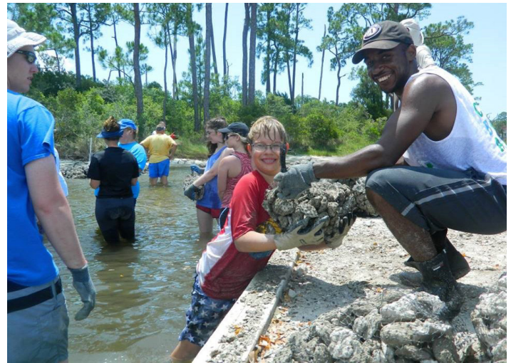
Figure 4. For living shorelines projects, oyster shell must be contained using mesh bags.
