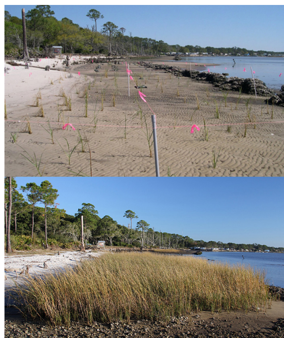
Figure 1. Living shorelines use natural materials like salt marsh grasses to prevent coastal erosion. In just four years, the progress of a living shoreline project in Franklin County, FL is substantial.
