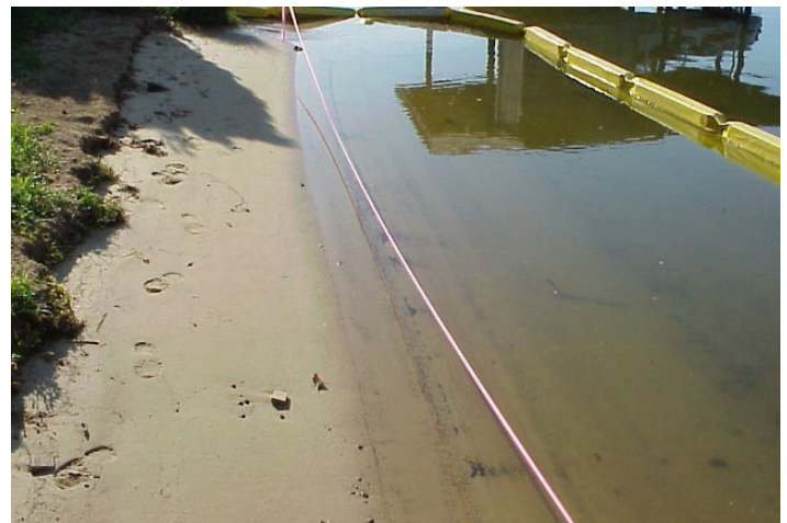
Figure 2. To qualify for a small-scale living shorelines permit exemption, the project must include plans to deploy a turbidity curtain to control silt and sediment.
