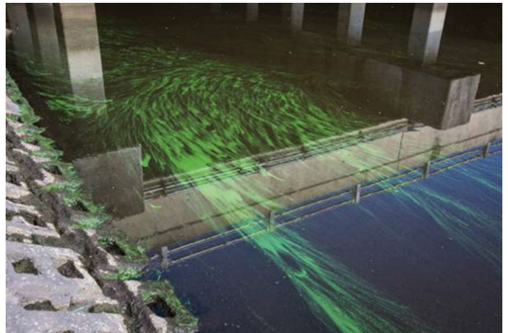
Figure 4. In summer 2016, the Microcystis from Lake Okeechobee was carried downstream in the St. Lucie River to the estuary. Here we can see water flowing under a highway bridge with bright green algae on the surface. The top edge of the bridge is reflecting in the water.
