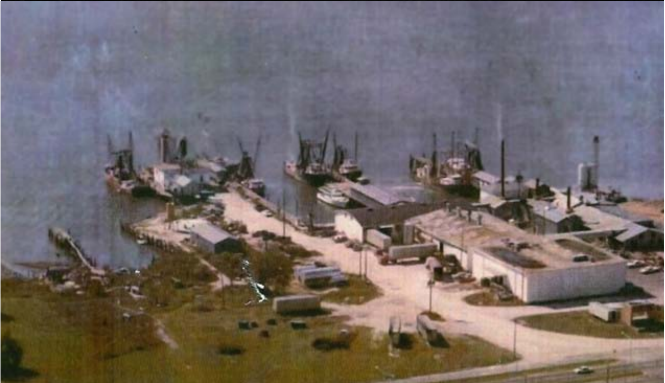
The Mavar factory in Biloxi, Mississippi prior to the expansion of the pet food processing building (top). The additional building was placed in the large open area in the left (west) of the photo at the head of the last dock. The bottom photo includes the additional processing building in the far right (west) of the photo.
