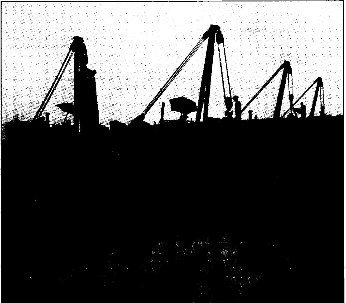
Laying a gas pipeline
