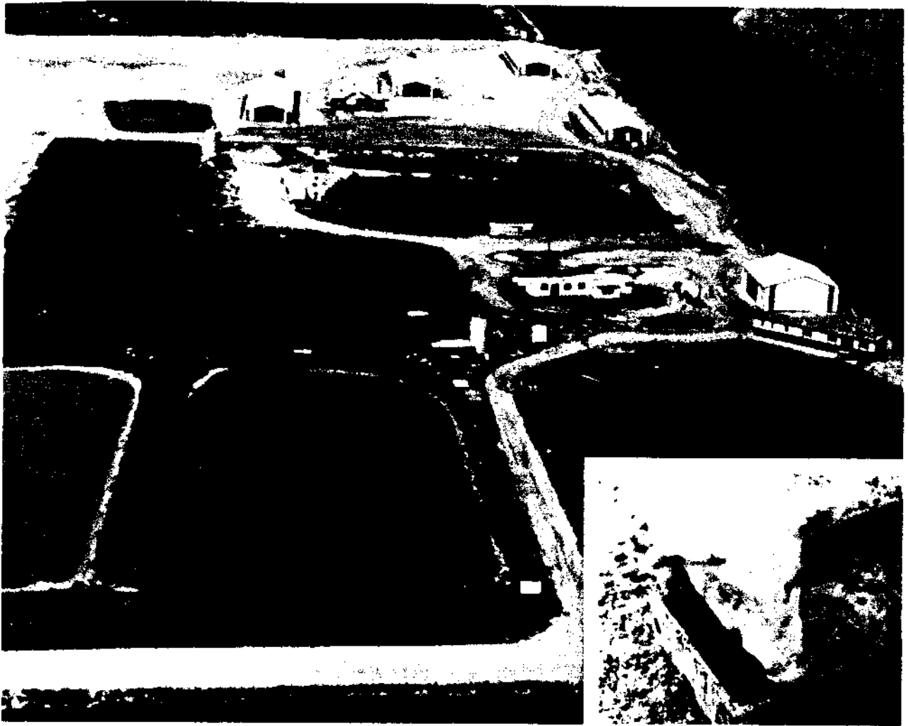
Figure 23. An algae production system using wastewater from a hog feed lot (Kansas). The resultant high protein algae slurry is the basic component of the hog feed (lower right). (Courtesy of M. Aitken, Algae Processes, Inc.)
