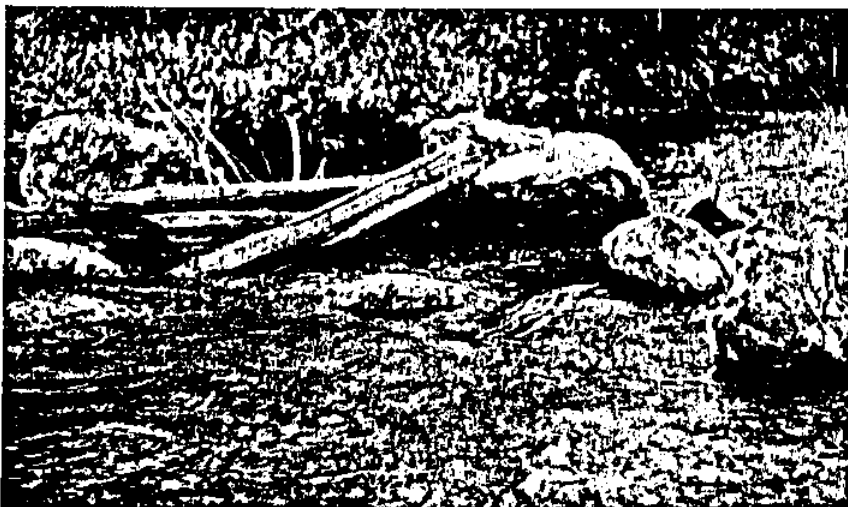
Appendix 3a. Three boulder grouping sites with log cover cabled tightly into the lead rock, increasing habitat complexity. Each boulder caused deepening of the site, but largely maintained the turbulent surface. This design was the most highly utilized by rearing salmonids and the most cost-effective.
