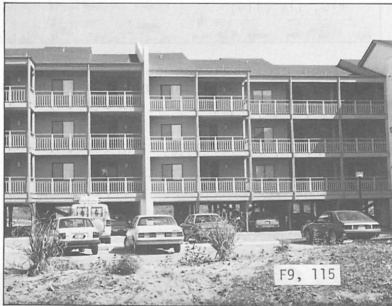
Figure 9. This example from Bogue Banks of a high rise condominium is typical of such structures built on pilings. The ground level is not counted in this three-story structure.
