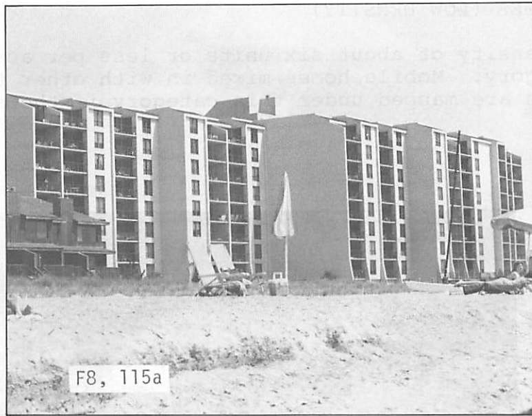
Figure 8. A ground view of the high rise condominium in Figure 7.
