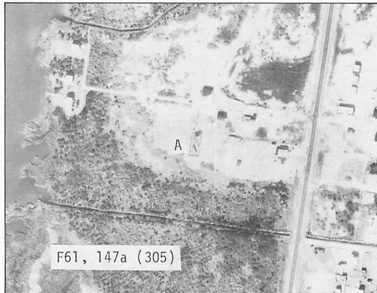
Figure 61. A power substation at Nags Head at point A. These skeletal structures are often difficult to detect on air photos because of their open nature. Sometimes the shadows of power line pylons and poles around the structure help identify it.
