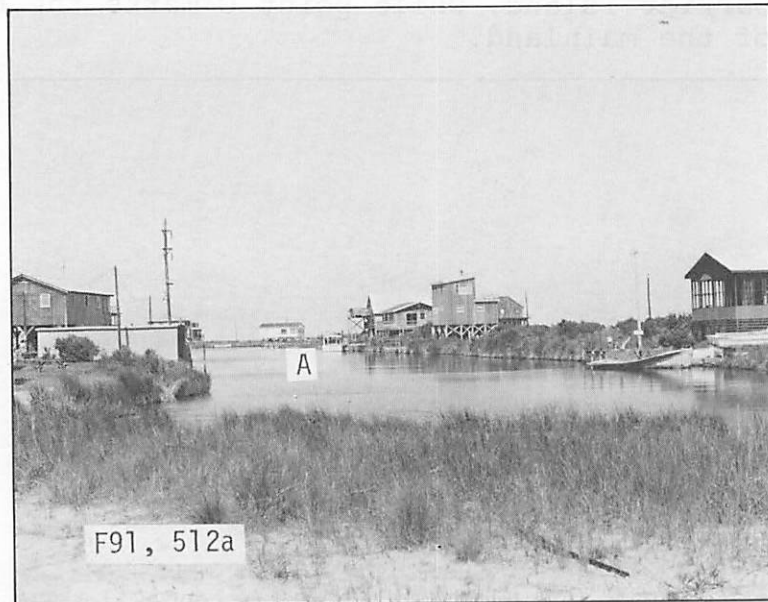
Figure 91. Spoil from the canal was dumped along both sides to raise the levels of the cottages being built there.
