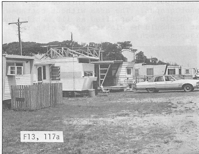
Figure 13. A typical mobile home high density situation on Bogue Banks at Salter Path. This is a view of point A in Figure 12.
