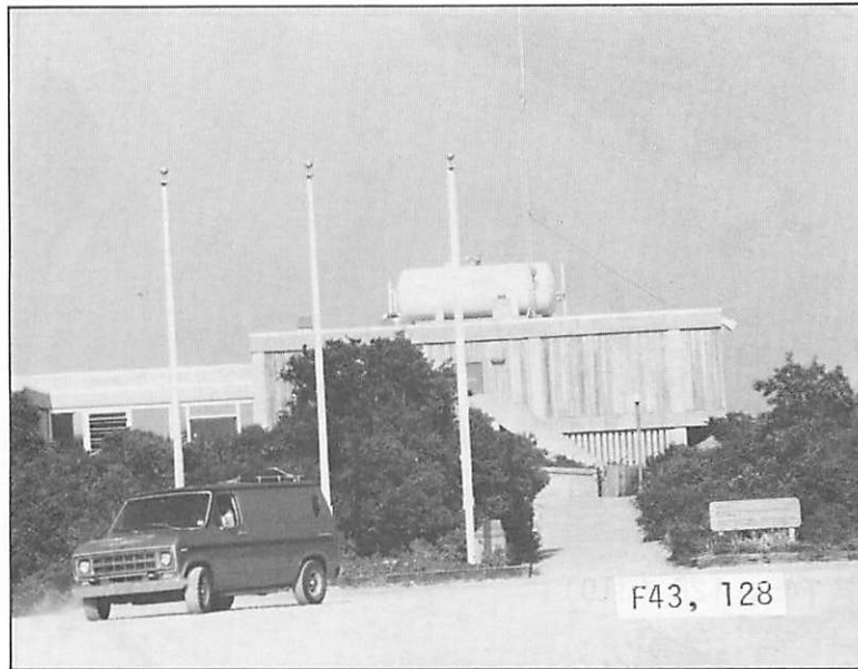
Figure 43. The Marine Resources Center at Fort Fisher. This is an institutional structure standing alone with its own parking lot.
