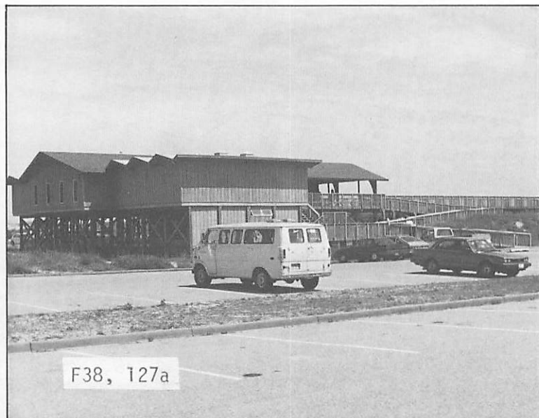
Figure 38. A ground view of the bath house and parking lot shown in Figure 37.
