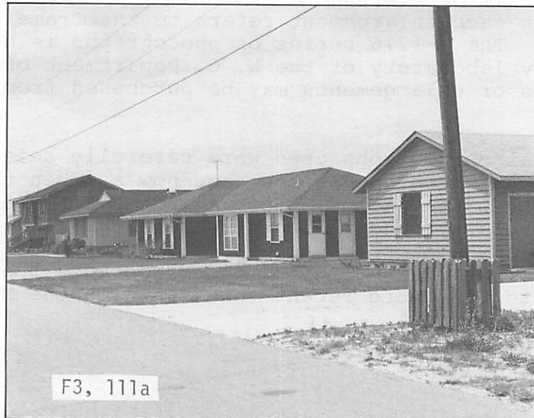
Figure 3. Ground view of single-family cottages at point A in Figure 2.
