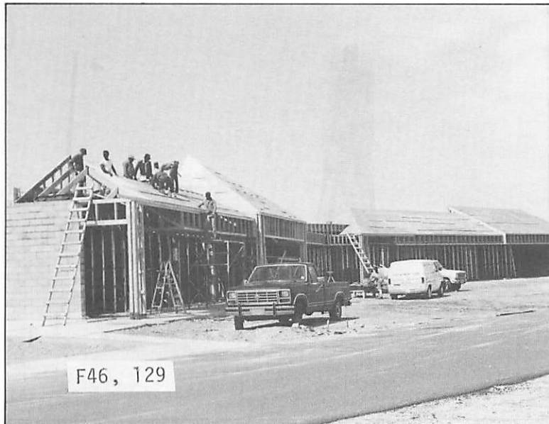
Figure 46. New stores under construction at Nags Head.
