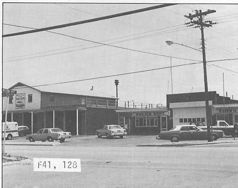
Figure 41. Town government buildings at Atlantic Beach. These would be difficult to distinguish from some commercial structures of category 122.
