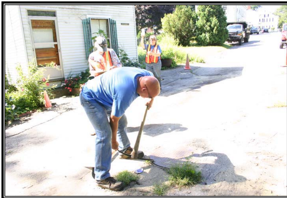
Figure 3 City of Dover Employee opening a Storm Drain for Volunteers
