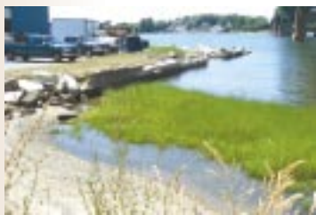
Sakonnet Bridge Access
