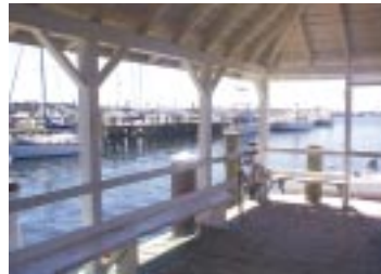
Ann Street Pier
