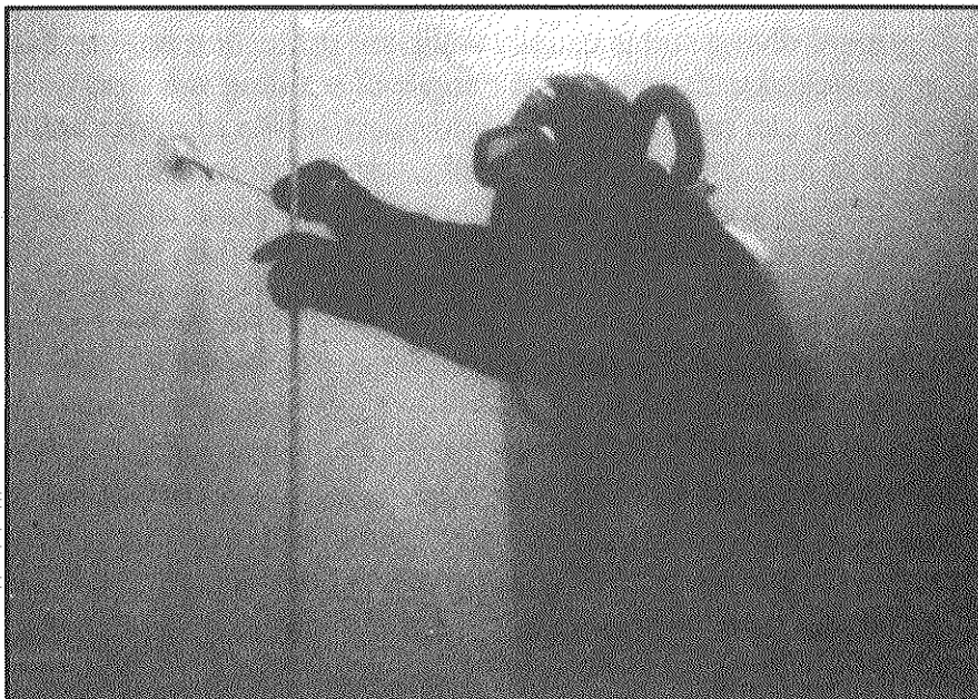
Photo 9: Diver working on the supporting wires around the plastic walls of a fish farming cage. Photo: Crown Copyright. Aberdeen Marine Laboratory
