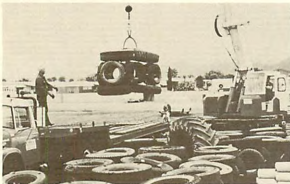
Local volunteers loaded and systematically placed these tire modules off the Ventura County Coast to enhance local fisheries.
