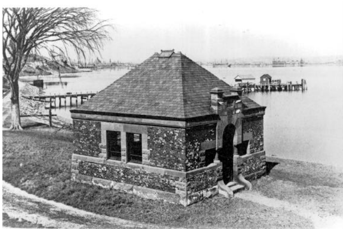
Plate 11 Outlet chamber for sewage discharge at Fields Point. From the 1893 annual Report of the Providence City Engineer.
