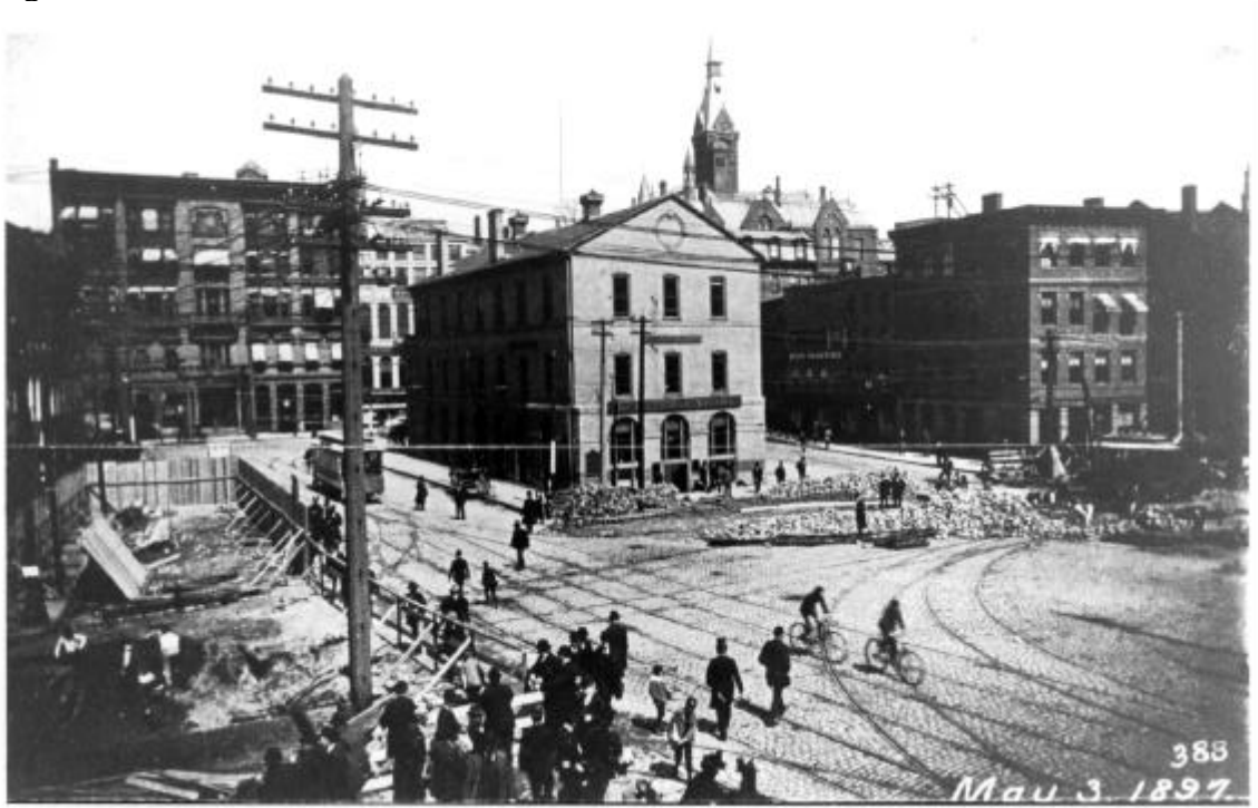
Plate 7 Paving streets in Providence with stone blocks in 1897. Sewage construction is also underway on the left of the upper photograph. Photos from the Providence City Engineer's office.
