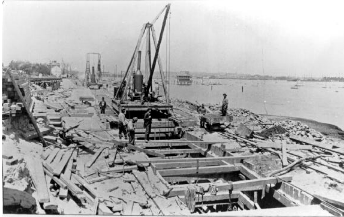
Plate 10 Excavating and plank driving machinery involved in sewer construction along the Providence River above Fields Point. From the 1894 Annual Report of the Providence City Engineer.
