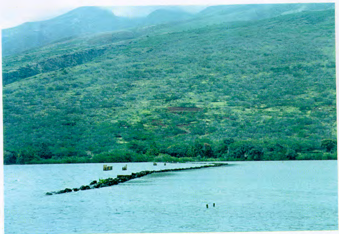
Fig. 1b Damaged wall of Keawaniu pond
