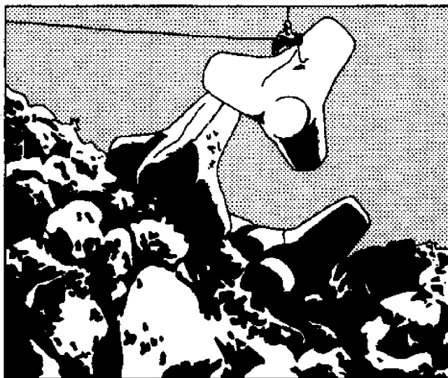
Placing first layer of tetrapods on rock embankment for a breakwater
