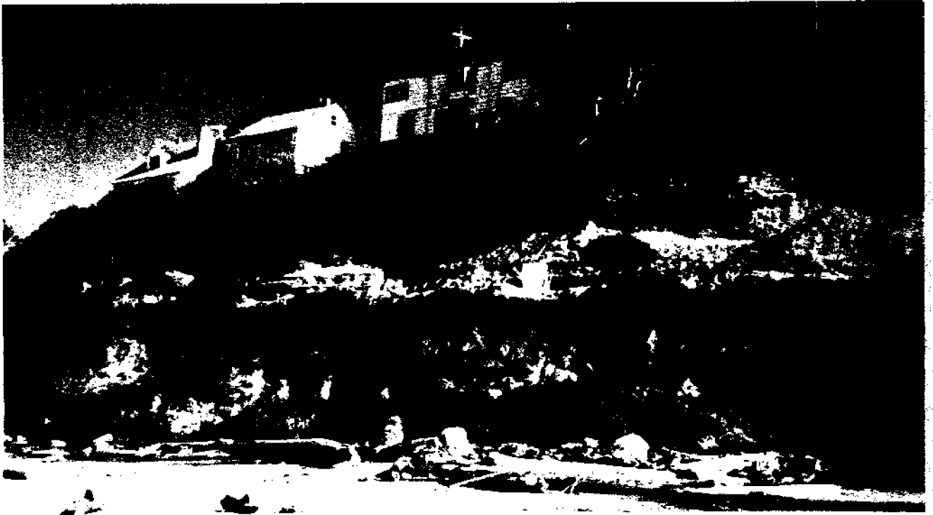
Figure 6: Sea-cliff erosion in Lincoln City threatening old houses and a new condominium.
