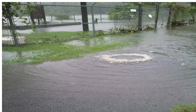
Roanoke Avenue Wastewater Pump Station - Hurricane Irene, August 2011
