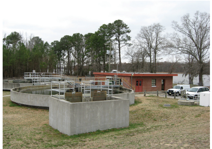
Portion of Plymouth's Wastewater Treatment Plant subject to flooding from the Roanoke River
