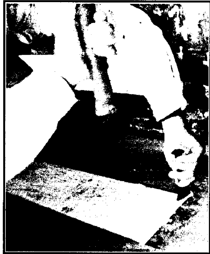
Figure 3. Caulking the hull
