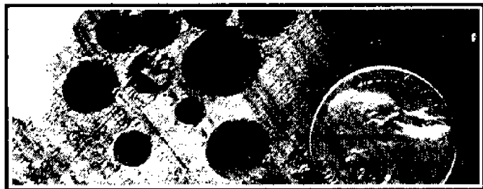
Figure 4 b. Damage caused by Teredo
