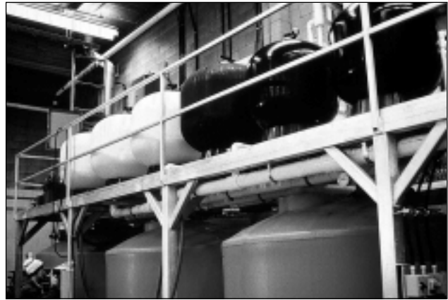
Figure 9. Mussel storage system, Vancouver, B.C. The big reservoirs (bottom) hold water for delivery to the storage tanks in Fig. 8. Above them is a battery of filtration units. This system uses UV to help control bacteria (David Scarratt photo).
