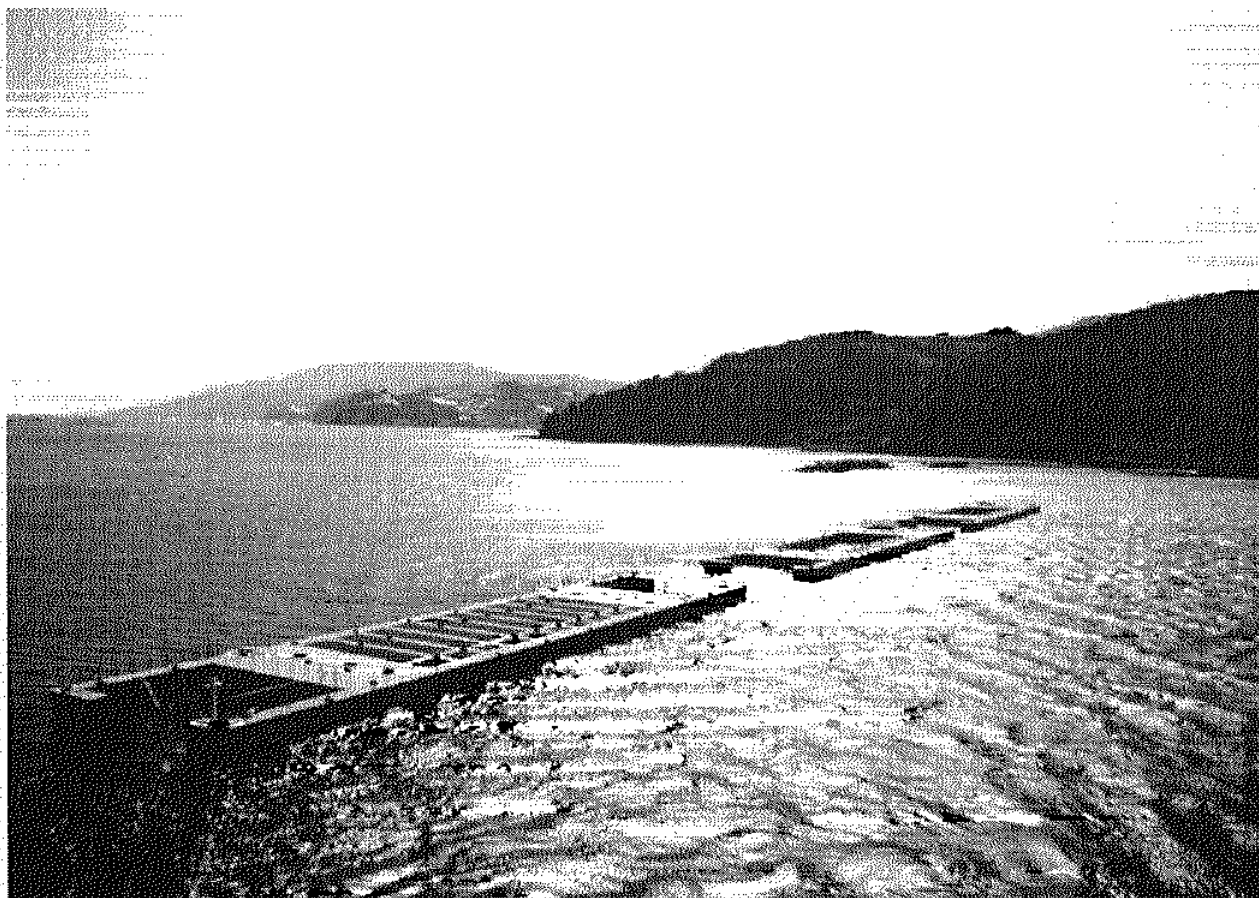
Figure 6. The floating breakwater
