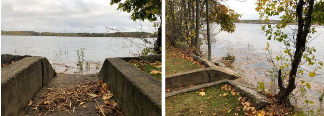
Extreme high tide at the stormwater outfall on Gulf Ave, into the Seekonk River. The tide measured 1.9 feet above mean higher high water—the projected sea level in around 15 years (D. Everett, 2020).
