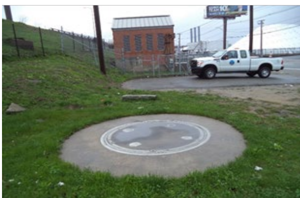
Improvements reduce vulnerability to the system. A flood protection door at NBC gate structure (top); watertight flood protection doors at the gate and screening facility (middle); and a water-tight utility vault/manhole cover (bottom) (NBC).
