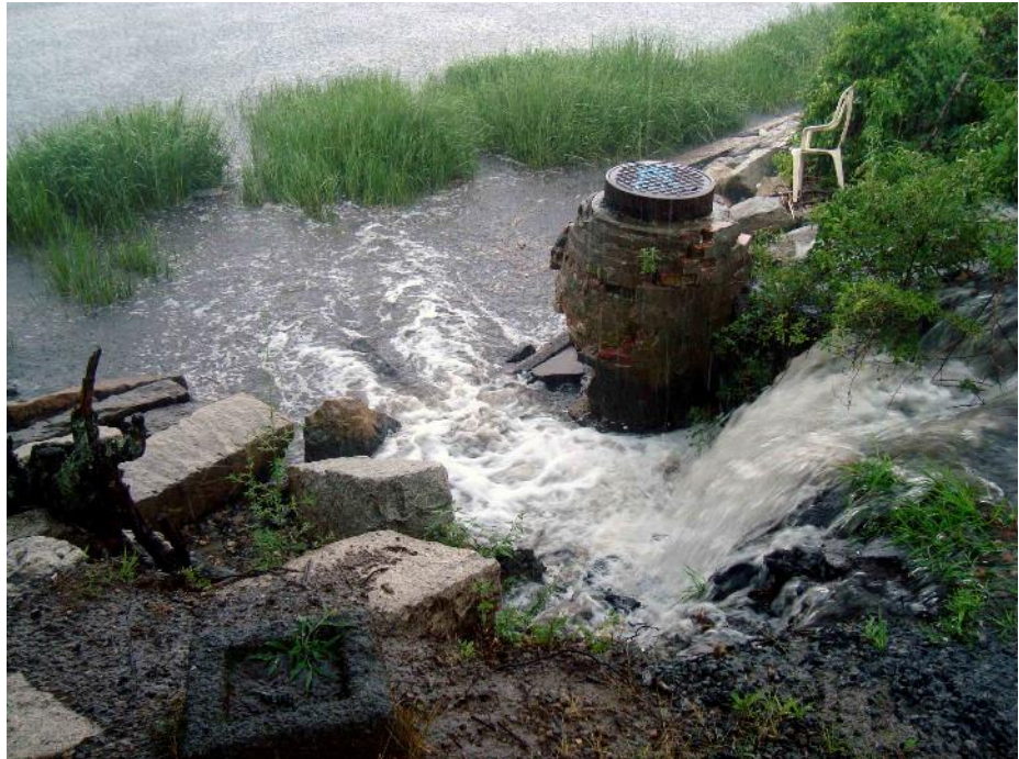
Infrastructure impacted by upland flooding on River Drive, Seekonk River. Upland flooding flowing down Irving Avenue has eroded the bank. Restoration is planned with grants awarded to the City (D. Everett, 2015).
