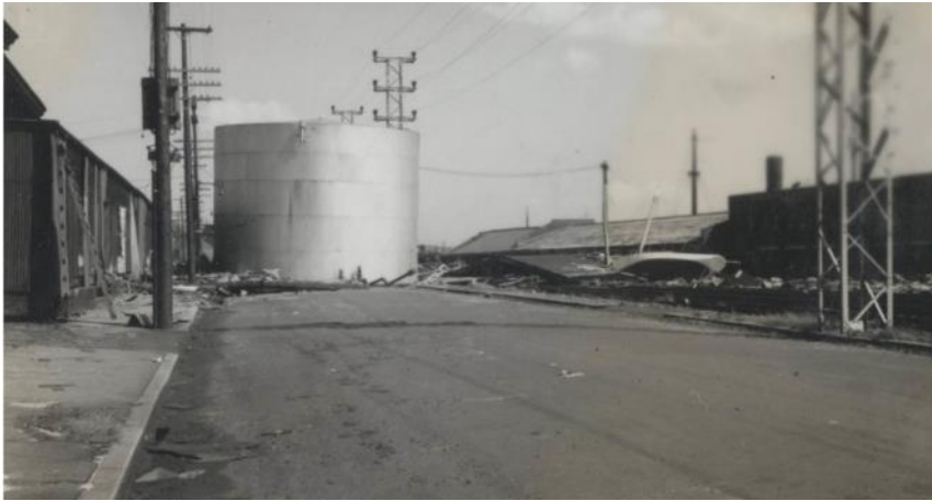
An oil tank floated to the center of the road by the 1938 Hurricane Storm Surge in East Providence (NOAA).
