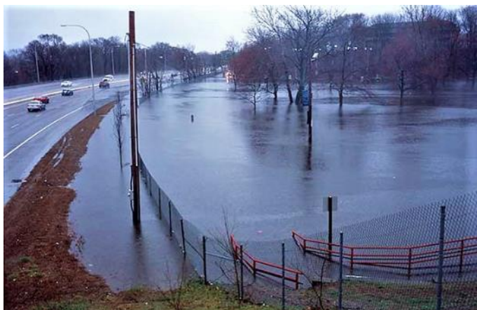
View of Merino Park from the Sheridan Street Footbridge during the 2010 Floods (A. Lehrer).
