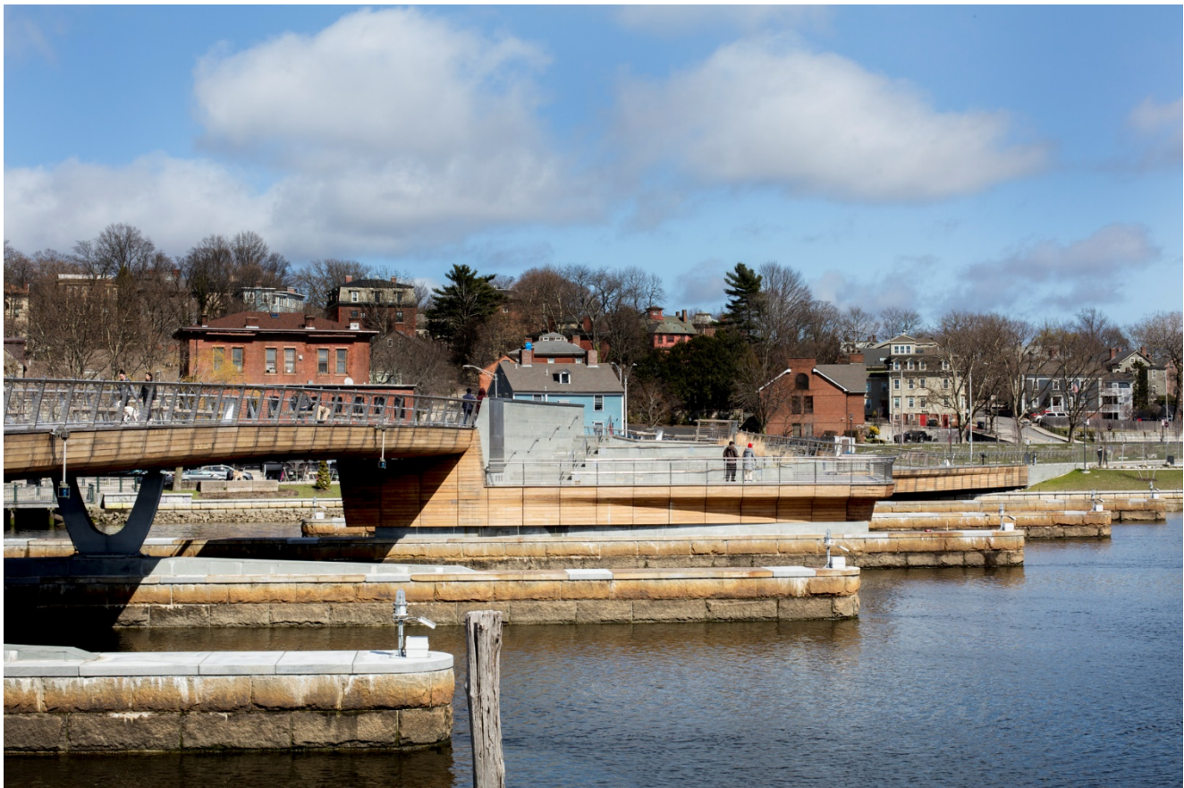
The pedestrian bridge design incorporated three feet of additional height to accommodate rising sea levels (K. Davis).
