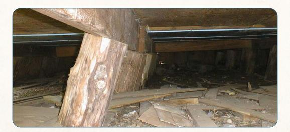
of adhesion, (as could easily happen in an earthquake. Better yet, if you are using dimensional or rough-cut milled lumber for your beams, use metal strong ties that fit so that you can nail or screw the galvanized tie to both the vertical supporting beam, as well as the joist(s) or beam above.
