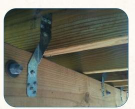
load path connection. In particular, the weakest link in most houses, the roof-to-wall connection, can be fortified with hurricane clips. You can install the hurricane clips after consultation with a licensed structural engineer or architect, or you can hire a licensed contractor who has experience in this area. Other portions of this work, unrelated to the hurricane clips, will most often require the work of
